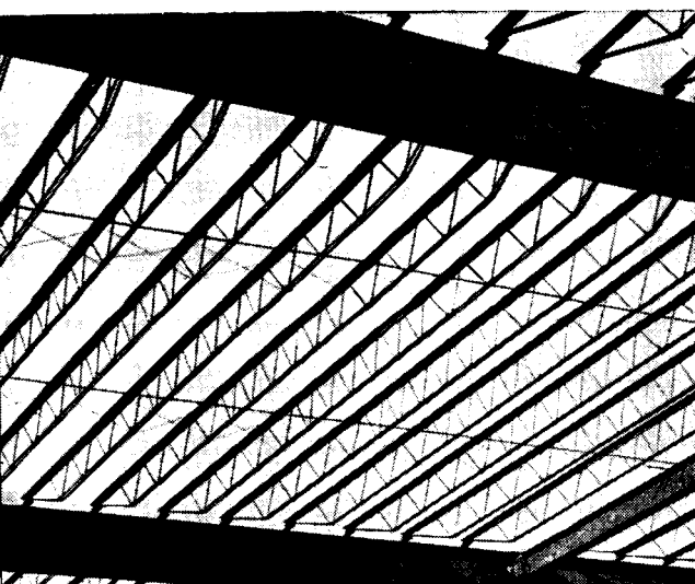
city of construction is made possible by Ceco steel joists. No needed in placing them. They are easily moved into position quickly spaced. After bridging, floor and ceiling are installed.
