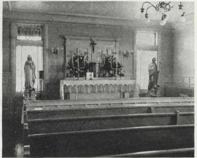
Chapel of Our Lady's Haven equipped with Automatic Sprinklers
