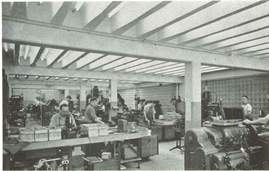
3. Structural elements serving as lighting fixtures illustrate design possibilities. (Installation at W. M. Welch Manufacturing Co., Chicago)
