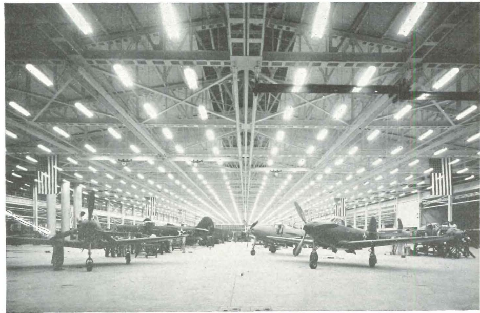
4. In a large interior, with high ceilings, the fixtures should be hung as high as possible. (Bell Aircraft plant, designed by the Austin Company)
