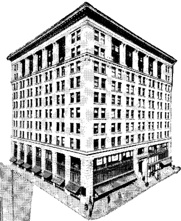
Slater Building, Worcester, Mass.
