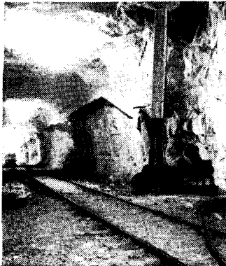
1 GYPSUM MINE. One of 9 National Gypsum deposits which insure a constant supply of selected gypsum rock.
