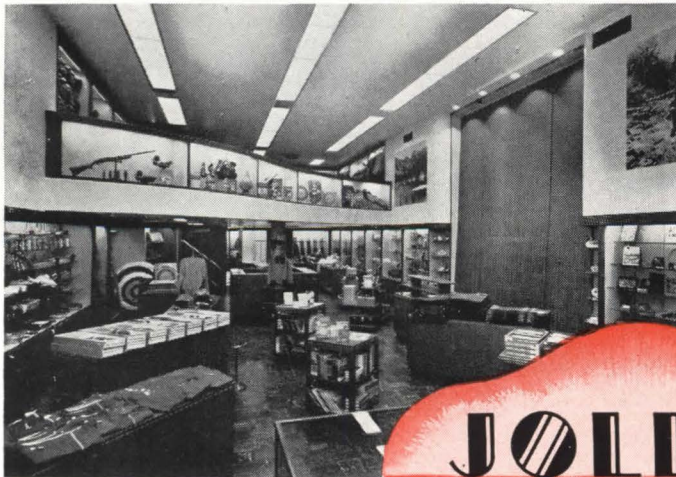
In the first floor main selling area, Joleco Slimline Fluorescents bring more than 70 footcandles of light to the merchandise level. Above and below the mezzanine 50 footcandles is maintained. Showcase fluorescents by Joleco increase selling effectiveness.
