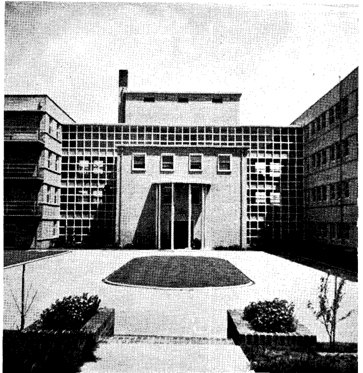
The Nurses' Home (right) also uses the system of prefabricated concrete frame, which lends itself to a variety of treatments — solid wall, windows, doors, ventilator or void
