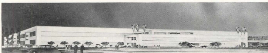
New Chevrolet assembly plant has concrete and glass exterior walls, concrete louvers
