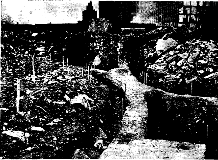
Old, hidden foundations of demolished gas tanks necessitated special pile-driving operations at Stuyvesant Town site. Beneath broken stone rip-rap lies concrete floor, 2 ft. thick
