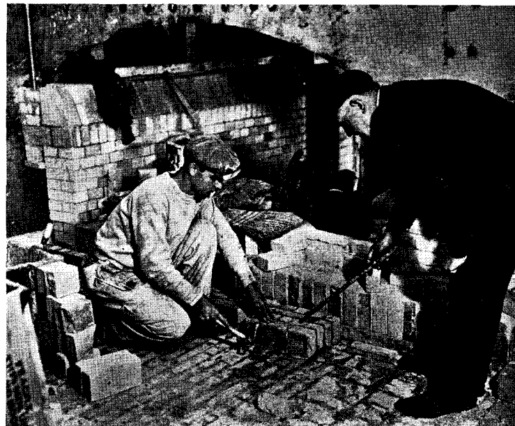
How to lay brick properly in a soaking pit floor is shown to apprentice Harry Floyd by H. D. Tyson, in a plant of the Tennessee Coal, Iron and Railroad Co. (U. S. Steel) in Birmingham, Ala.
