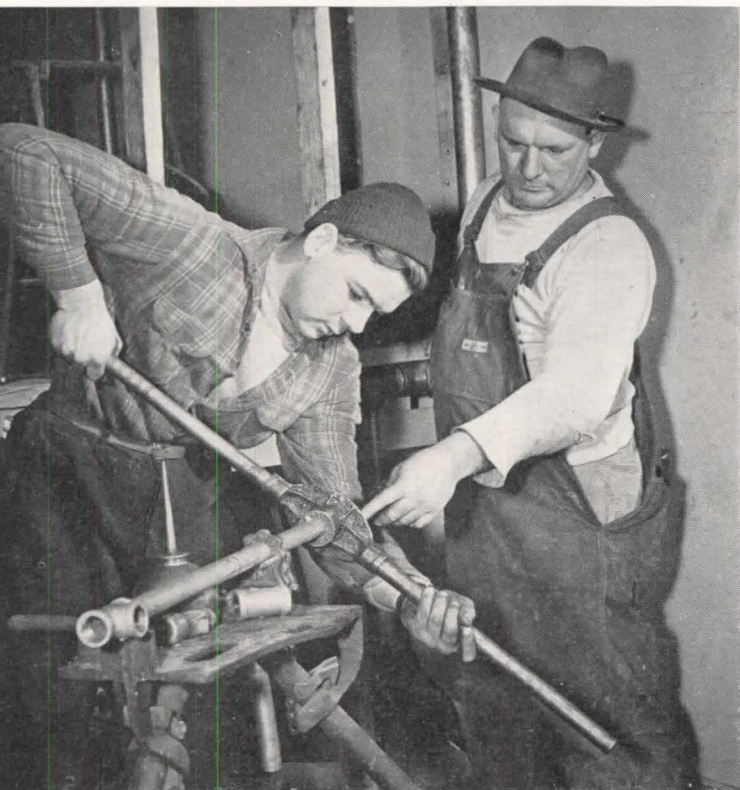
The tradition of craftsmanship is here being carried on by a father-and-son team. Journeyman plumber John E. Grove of Washington, D. C., shows John G. Grove how to thread a pipe
