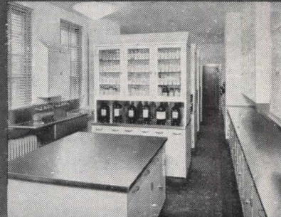
A BRIGHT, ATTRACTIVE pharmacy. Sink, table tops and counter tops are Monel.
