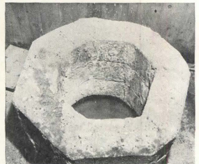
The sump pump well is no longer used. Pump was disconnected months ago. Water still rises to the floor level as can be seen in the above photograph—proving that the floor and walls of the pit are still surrounded by water held back by Aquella.
