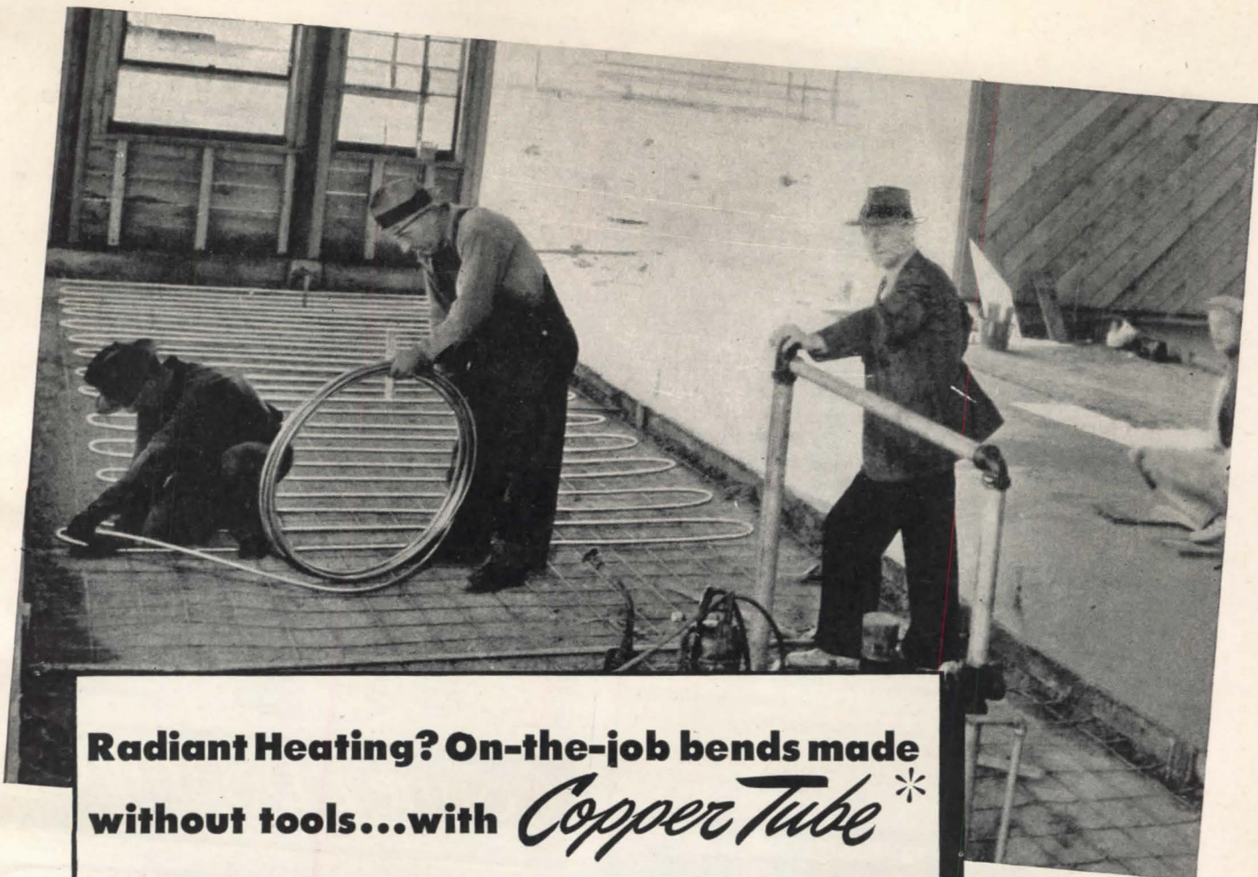
Radiant heating installation of Copper Tube in San Leandro (Calif.) sterilizer factory. Installation by Robert Bruen & Son.
