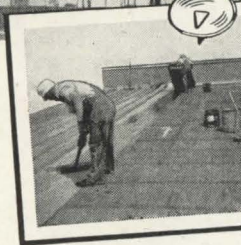
Generating station, Northern Indiana Public Service Co. Supplies electric power for 229 midwest communities. Right: Workman applies protective Abesto coating.
