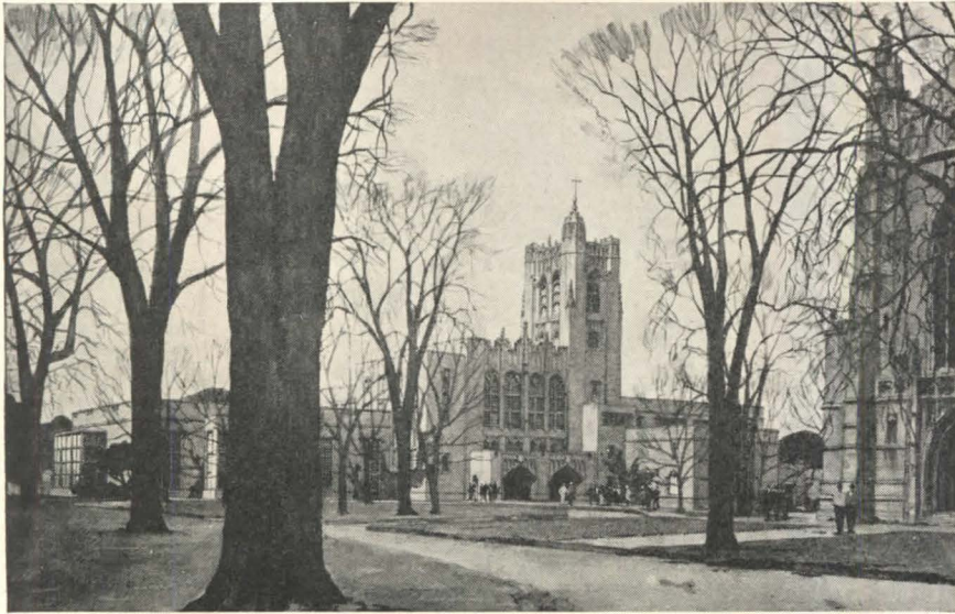
Princeton University's new library, scheduled for completion in June, '48. R. B. O'Connor and W. H. Kilham, Jr., Architects. (See ARCHITECTURAL RECORD, Jan. '47, pp. 99-101)
