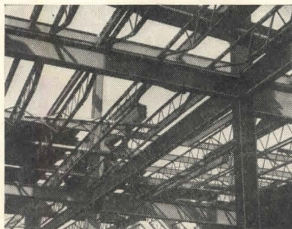
Truscon Structural Steel in Armstrong Plant
