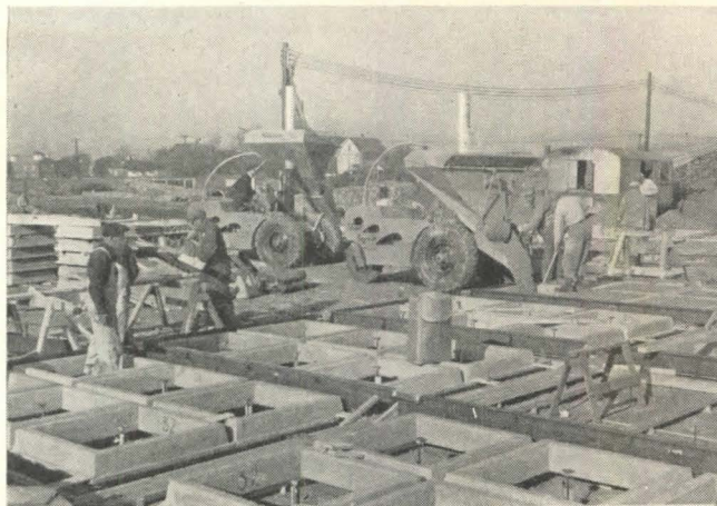
Steps in casting the concrete mold. Left: Precast hollow squares are placed within metal edge forms and blocked above the ground. Abutting flanges of the squares will form the mold for the ribs of the slab. Compressed-air risers are set in the center of each square, and concrete poured flush with their cover plates. Right: Completed mold after surface has been finished and reinforcement set in place
