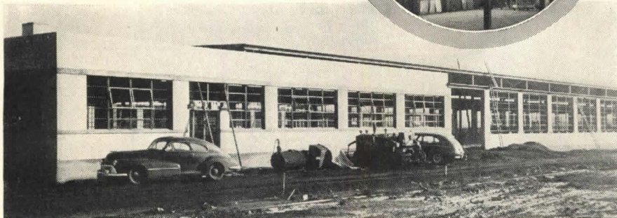
Exterior View of the Armstrong Furnace Company, Columbus, Ohio, Showing Truscon Architectural Projected Windows in Office Building.
