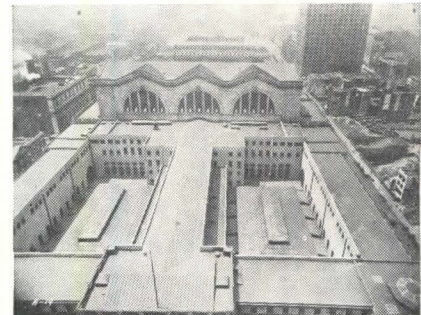
37 YEARS YOUNG. This batten type Monel roof on New York's Pennsylvania Station covers an area of 300,000 square feet. It was installed in 1910, shows no visible signs of deterioration today.
