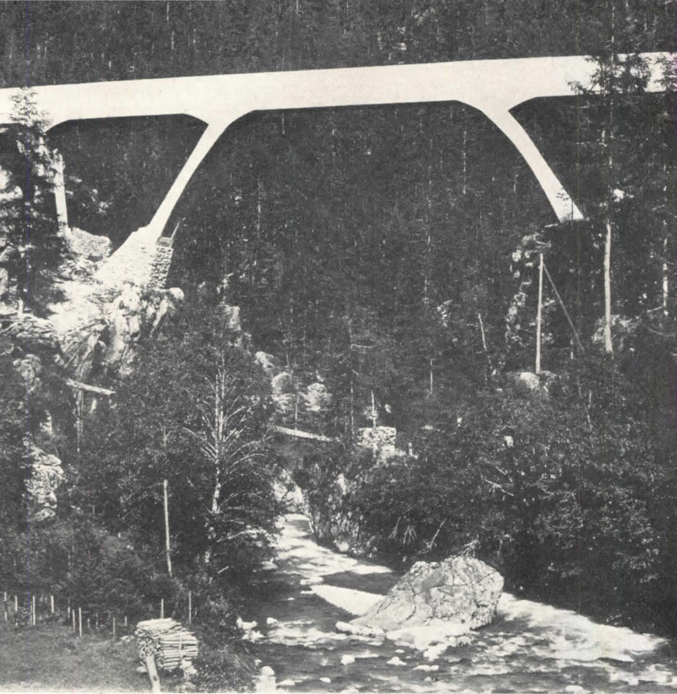
Left: Chatelard Aqueduct (1925-26), Canton Valais. In this structure, the arch starts its spring from the abutments with more or less orthodoxy, to fuse in mid-span with the box girder which itself, economically, carries the water. Above:
