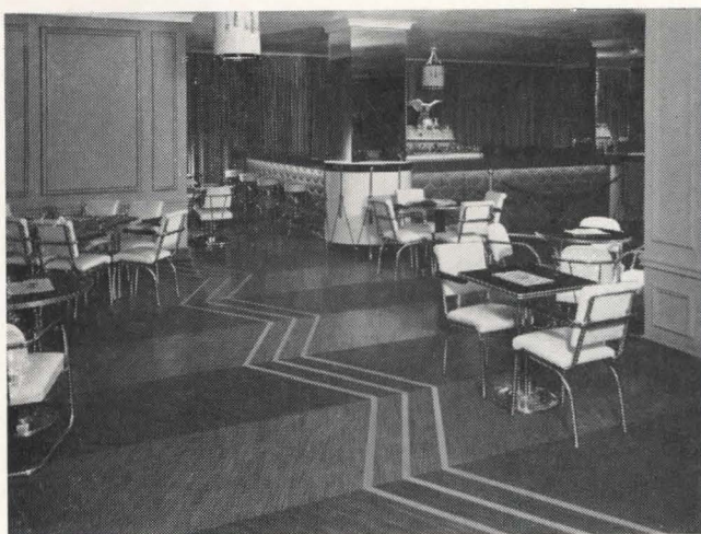
Resilient flooring material gives the architect many opportunities to carry out the theme of the interior in the floor design. Here the military motif of the room's decorative scheme is picked up in the stripe and chevron design of the floor. Two colors of jaspé linoleum form the stripes, while plain linoleum was used in the rambling chevron design.
