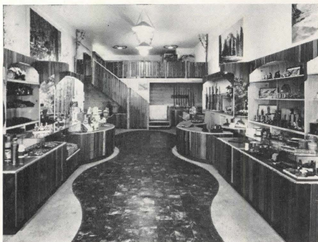
While geometric designs are the most commonly used in custom floors of resilient tiles, sweeping curves, scrolls, and similar designs can be executed equally well in asphalt tile, Linotile®, or rubber tile. The picture above illustrates how an attractive asphalt tile floor can be custom designed to follow the curved contours of the interior layout.
