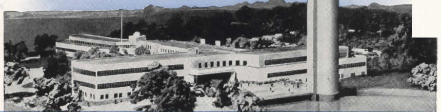
Federal Telecommunications Laboratories, Nutley, N. J. Largest all-metal commercial group in the world. Architects—Louis S. Weeks, N. Y. C. (groups 1 & 2); Giffels & Vallet, L. Rossetti, Detroit (groups 3 & 4).
