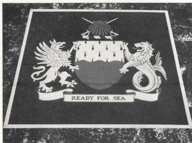
This elaborate floor inset reproducing the Marine Air Insignia is a typical example of the unlimited decorative possibilities of resilient flooring materials. Eight colors and more than two hundred individual pieces of asphalt tile were used in the inset which was cut to designer's specification and shipped as a complete unit from the Armstrong factory.
