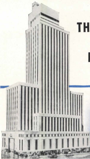
Mercantile National Bank, Dallas, Texas. Tallest office building in the South. Architect—Walter Ahlslagler, Dallas. Contractor—Henger Construction, Dallas.
