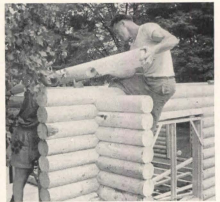
Ready-made logs aid rapid construction
