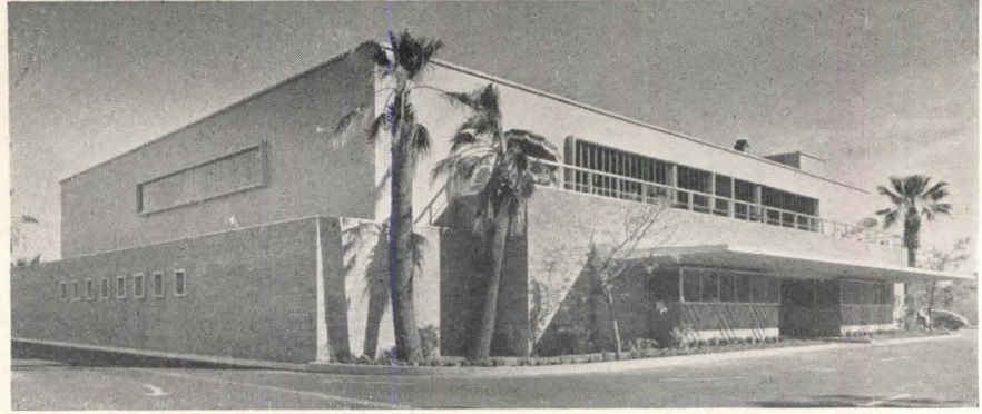
Another view (the parking entrance) of Bullock's Palm Springs store, shown in detail on pp. 123-127 of the April RECORD. Walter Wurdeman and Welton Becket, A.I.A., Architects
