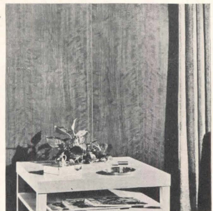
Simulated walnut finishes are reproduced on a base of Presdwood for wall panelling
