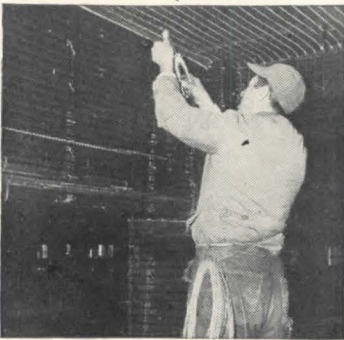
PLIABLE AND EASY-HANDLING. Monel Tie Wire is solid, ductile. Has no coating that flakes off when bent. Twists to a snug fit without breaking.
