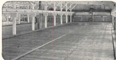
Group Lift Saves Labor on Ice Tanks
