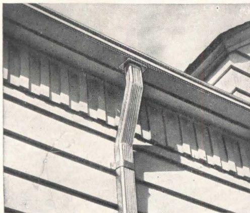
DOWNSPOUTS: Roof drains that will last forever—that's the dream stainless steel makes come true. The downspouts pictured here have been up 10 years.
