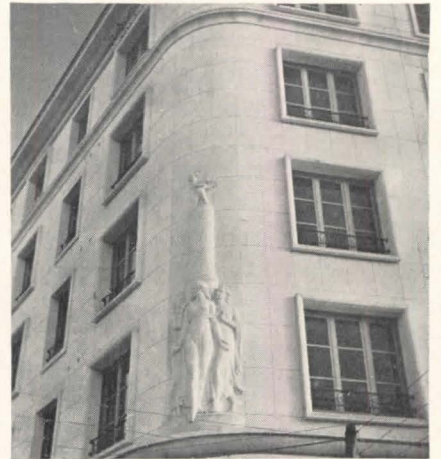
Left: one of the Orléans apartment units built by the "prefabrication-montage" procedure. Below: corner of one of the buildings, showing the sculptured figures by Poisson
