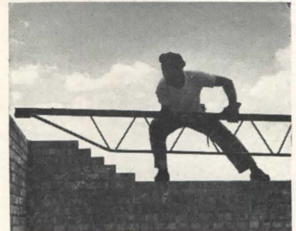
FASTER —Ceco Open-Web Steel Joists are light and easy to install. Special equipment and falsework are unnecessary. This results in speedy erection and minimum interference with other building trades on the job.
