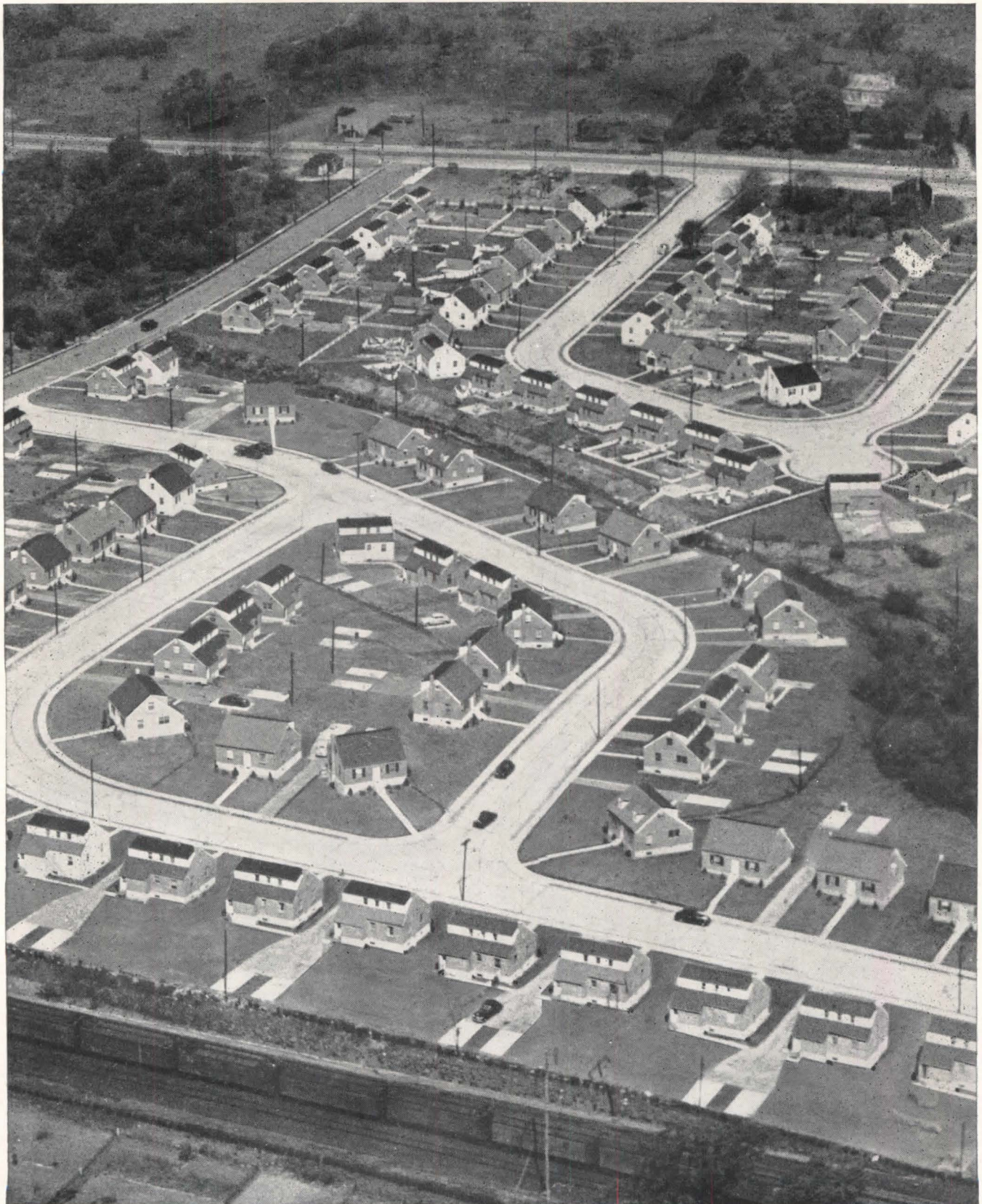
Steel Joists in Housing Project — Located in Sharon Hill and Folcroft, Pa., this well-planned development is known as Sharon Park. It consists of 114 two-story-plus-basement brick homes. Bethlehem Open-Web Steel Joists are used in the floor constructions of both the first and second floors, where they are combined with concrete slab and plaster ceilings. This floor construction is not only economical, but makes these homes fire-safe, as it prevents fire from spreading for a period of at least two hours. In addition, it is shrink-proof, sound-retardant, and immune to attack by vermin. Architect: S. Arthur Love, Jr., Norwood, Pa. Contractor: Donald M. Love, Norwood, Pa.
