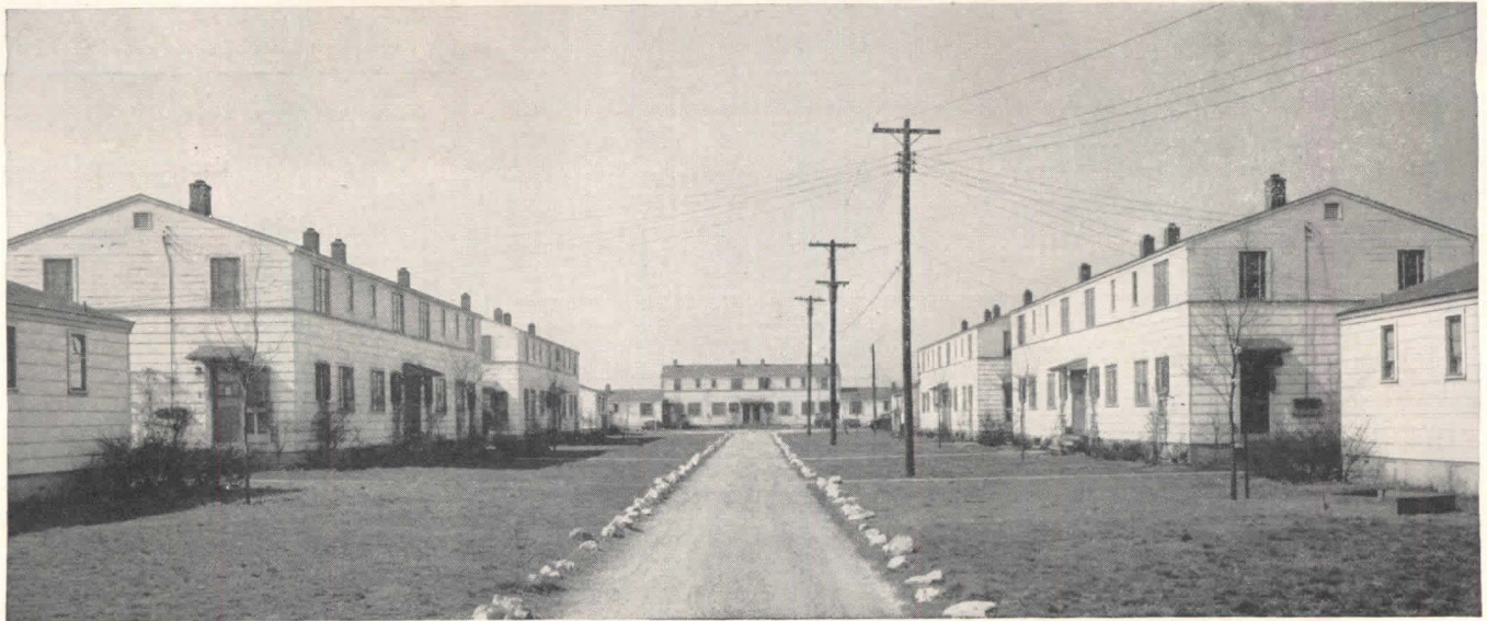
This Indiana housing development features "Century" Asbestos-Cement Siding on first stories, with K&M "Century" Apac board used as skirting at the foundations.
