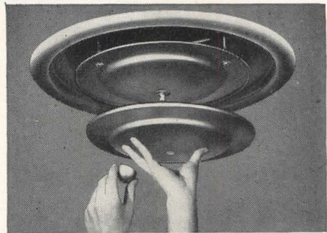
Step One: Remove cover cone (if used)
