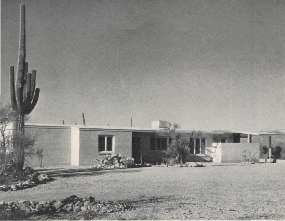
A new bedroom wing will extend out from blank wall at left in this photograph; entrance to house from carport, at extreme right, is through the walled service yard. Roof is built-up composition over 4-in. mineral wool insulation
