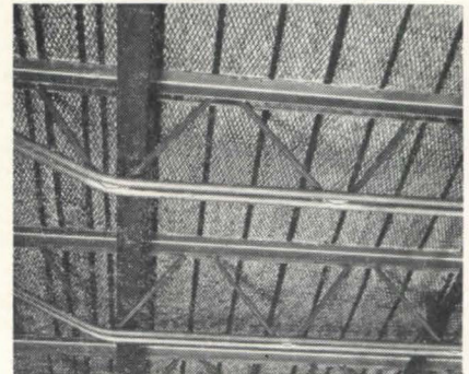
ECONOMICAL —Ceco's Open-Web Steel Joists are self-centering. The form work for the concrete slab—usually metal rib lath or steeltex—rests directly on the steel joists without other support from the under side.
