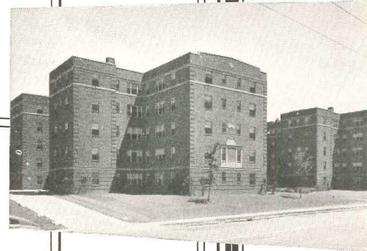
Kemper Road Apartments, Cleveland, Ohio. Truscon 138 Double-Hung Steel Windows used throughout. Weinberg, Laurie & Teare, Architects. Charles Bernstein, Builder
