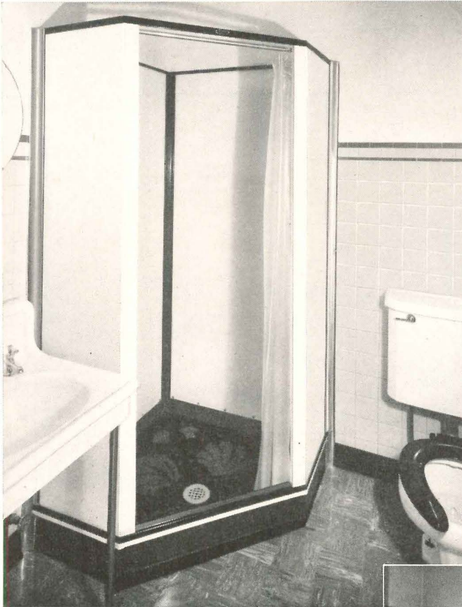
Before and After Modernizing bath- rooms in Hotel Van Orman, Fort Wayne, Indiana.
