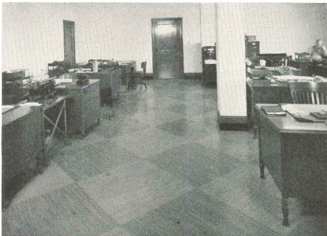
The office area above illustrates one of the many decorative effects possible with jaspé linoleum. The alternate square design used here is ideal for both large and small areas since the jaspé squares can be cut to any desired size. These effects can be worked out in related or contrasting colors.
