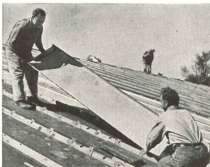
INSTALLING MONEL BATTEN PANS over wooden batten bars. The pans have pre-formed ends that provide watertight joints without solder. Monel nails and cleats are used to lock the pans and the Monel batten caps together.
