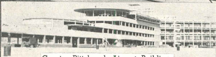
Greater Pittsburgh Airport Building
