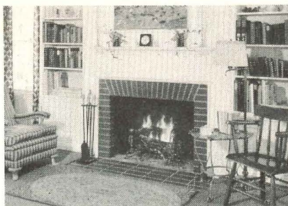
A Colonial Fireplace built around a Heatilator unit. Warm-air grilles are located in the bookshelf sides.
