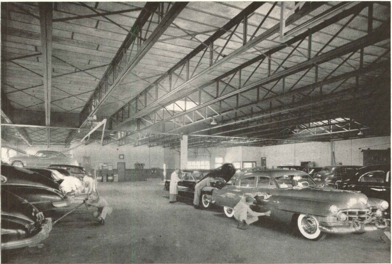
Bethlehem Longspan Joists in garage of Crossman Cadillac, Inc., Great Neck, Long Island
