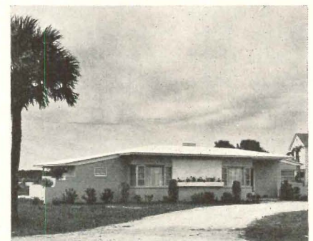
Light-colored marble chips over aluminum foil forms lightweight roofing with good reflective insulation values
