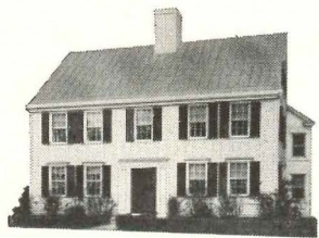
OLD NEW ENGLAND HOUSE Terne Metal Roof installed almost 100 years ago
