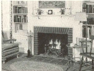
A Colonial Fireplace built around a Heatilator Unit. Warm-air grilles are located in the bookshelf sides.
