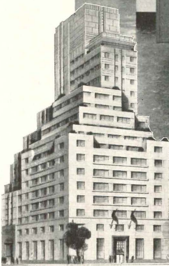
Crowell-Collier Building, New York, N.Y. Architect: Leonard Schultze Associates, New York, N.Y. Fixture Manufacturer: Miller Company, Meriden, Conn. Electrical Contractor: L. K. Comstock, New York, N.Y. Glass: CORNING ALBA-LITE in 2,600 Reflector Sections
