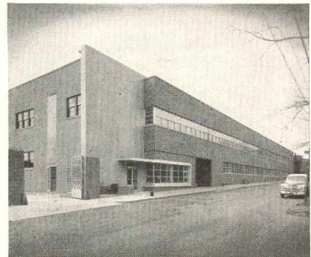
This modern warehouse and operating building of The Peoples Natural Gas Company, Pittsburgh, Pa. incorporates a steel pipe radiant heating system for warmth, protection of delicate instruments and even for snow removal.
