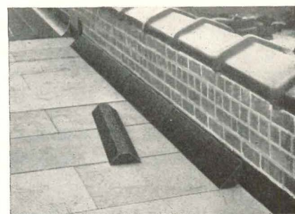
Cant strip of cane fibre board is lightweight, strong, easy to cut and handle
