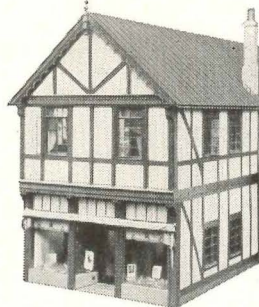
REPLICA OF MEDIEVAL ENGLISH HOUSE Design of Terne Metal Roof conforms to architectural treatment
