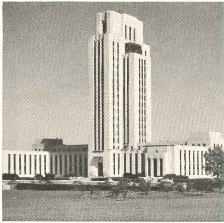
A total of 2200 Roddiscraft Solid-Core Flush Veneered Doors are in use at the United States Navy Medical Center in Bethesda, Maryland.
