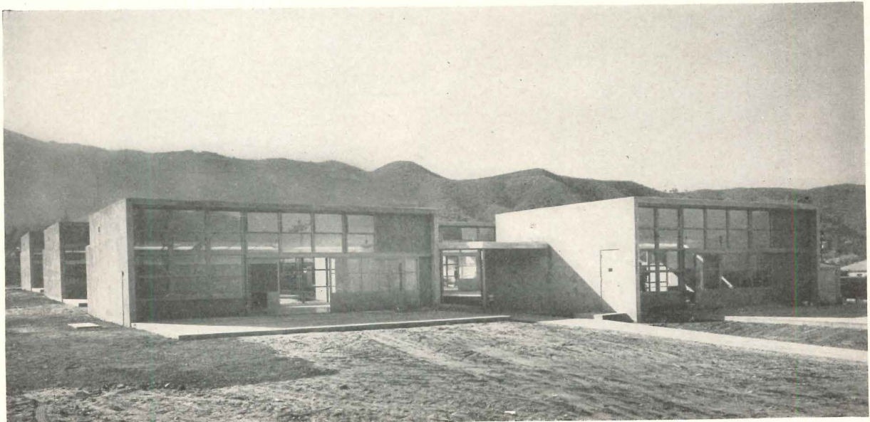
Classrooms at Apperson are staggered along a north and south corridor. Large ceiling louvers control light on south side; north has all-glass wall. Outdoor classrooms paved
