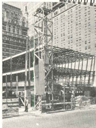
Truscon "Clerespan" Joists used in Adolphus Garage, Dallas, Texas.
