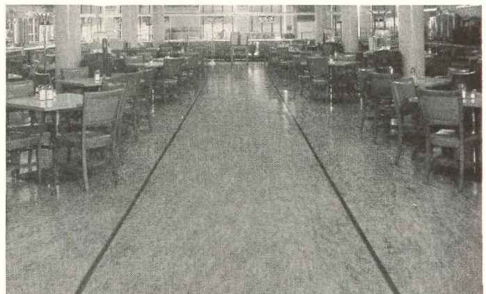
4. In the cafeteria of the American Furniture Mart, Chicago, Ill., linoleum is especially effective because its resilience assures both easy, quiet walking and sure footing for patrons carrying heavily loaded trays. Smooth, crevice-free surface insures cleanliness.
