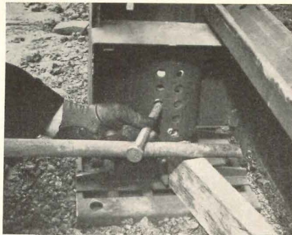
Photos at right show erection process. Footings (above) set on top of ground, are adjustable through a range of 3 in.
