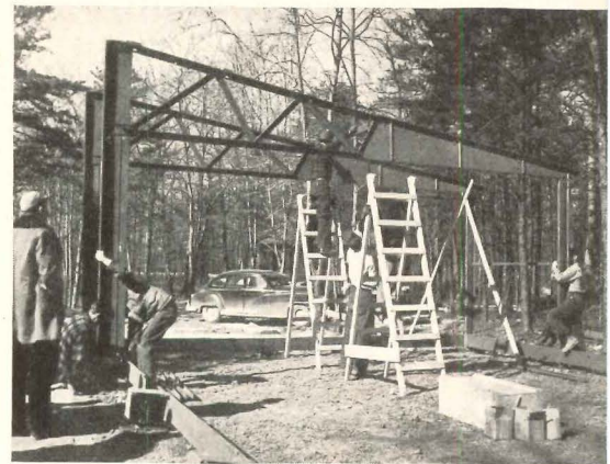
Photos at right show erection process. Footings (above) set on top of ground, are adjustable through a range of 3 in.
