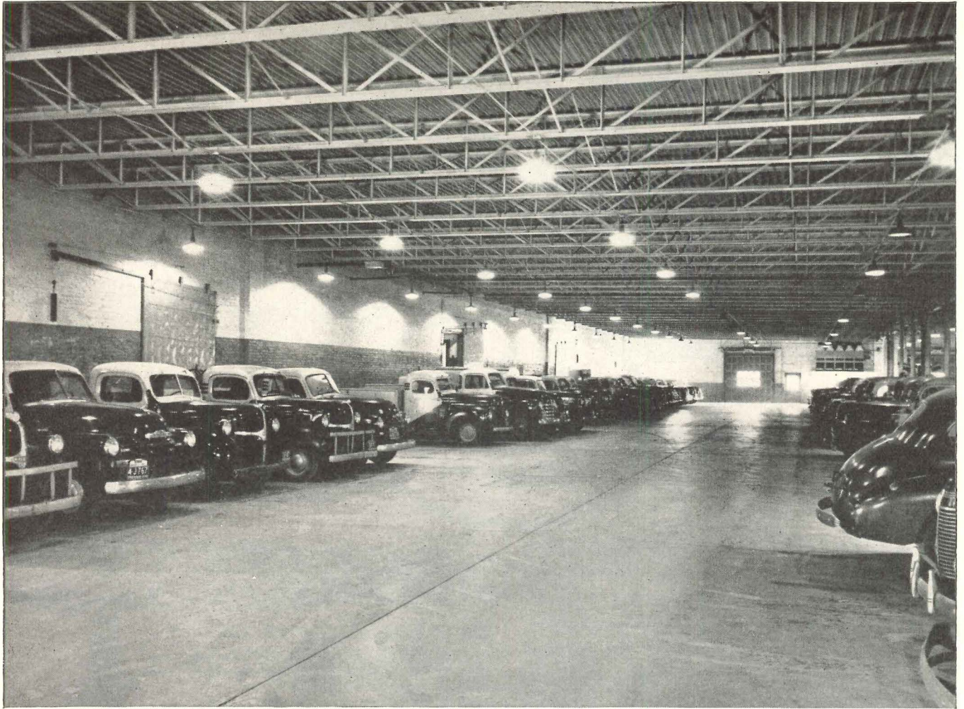
Bethlehem Longspan Joists in garage of Ohio Fuel Gas Co., Toledo, Ohio.
