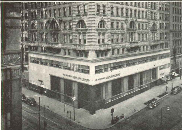
Extensive remodeling was limited to quarters for bank occupancy
