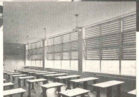
Stationary steel louvers were employed to control light, deflecting it to the ceiling.
