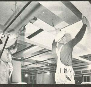
Standard 11/2" Metal Channel is Used for the "Grid"
