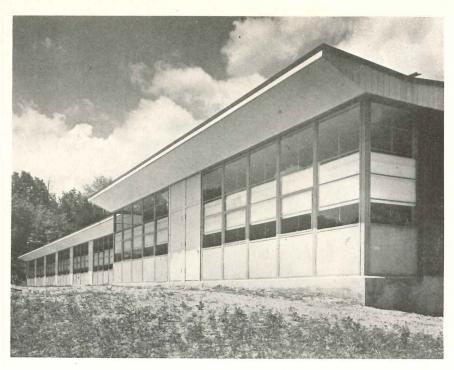
The classrooms face south and have doors to the outside. Sheets formed of insulation between asbestos cement layers form the wall below steel windows
