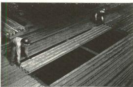
Raceways go in as the Q-Floor is laid, because—with G-E Q-Floor wiring—the floor is the raceway system. Each floor cell is a complete raceway, ready to receive wire, ready for electrical changes any time during the life of the building.
