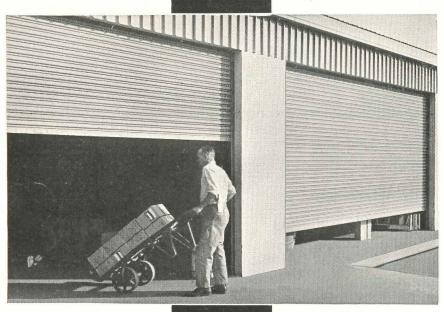
Low-Cost Repairs. Slats individually replaced if damaged.
