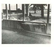
The complete unit may be obtained with frames of treated wood or extruded aluminum, and can be installed in frame or masonry walls or in construction combining both. Glazing may be single, double or triple plate glass. Heat loss is reduced by weather stripping and insulation. Both interior and exterior trim are furnished with the units, which are available in stock sizes or in made to order specifications. Solar Air-Flo, Inc., Dept. A., Elkhart, Ind.
