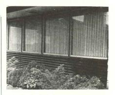
Window units with ventilators present simple louvers on exterior (above), tilt-out doors for air control on interior (below)
