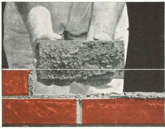
A good bond was secured here because the mortar was not sucked dry too fast.
