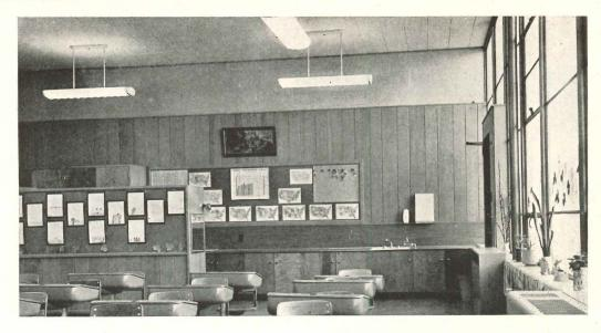
Views of two types of classrooms show pine vertical board wall finish, with exposed concrete block above; note use of cabinets at project areas. Below is typical end-wing classroom, this one a primary room furnished with tables and chairs
