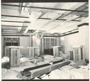
Metal Panels are Quickly and Easily Secured to "Grid" with Metal Clips—Perfect Alignment Assured. Acoustical Material Rapidly Positioned
