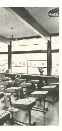
Note framing module based on steel sash and plywood sizes
