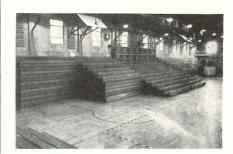
Folding bleachers are shown above in closed, partially open and open positions
