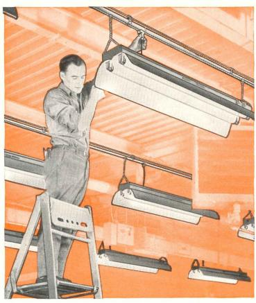
Safe, simple, quick! Tap off power from totally enclosed bus bars at any point along the continuously slotted duct with handy trolleys or twist-out plugs. Universal Trol-E-Duct both supports and supplies current to these fluorescent lighting fixtures.
