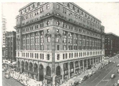
J. L. Brandeis & Sons, Omaha, has installed a Worthington 67C98 centrifugal refrigeration system (647 ton capacity) for air conditioning the lower floors of this store building. Engineering by Charles S. Leopold Company
