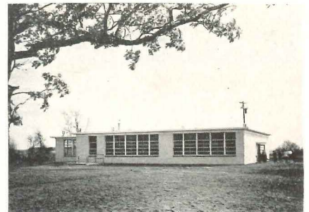
First unit of expandable school is equipped with heater to serve next addition
