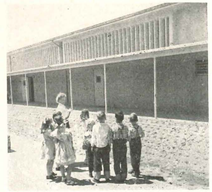
Vertical louvers in new school (above) are automatically operated by photo electric cell and motor. A single master louver controls the entire bank (below)
