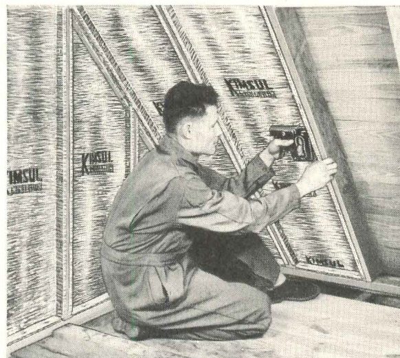
4 Flanges stapled to sides of framing hold blanket permanently in position and also provide air space. Part of flange folds over face of framing to complete vapor seal.
