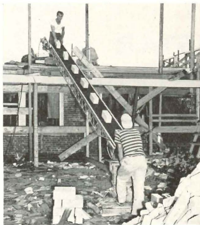
Conveyor simplifies and speeds transportation of brick to second floor levels
