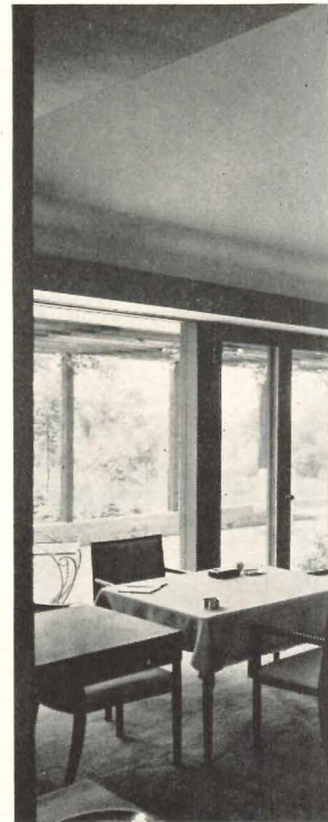
Clerestory above interior corner of living room admits light, ventilates, forms a plant shelf which, continued around two sides of the room, becomes an indirect lighting trough. Ceiling is higher in living room than in other rooms
