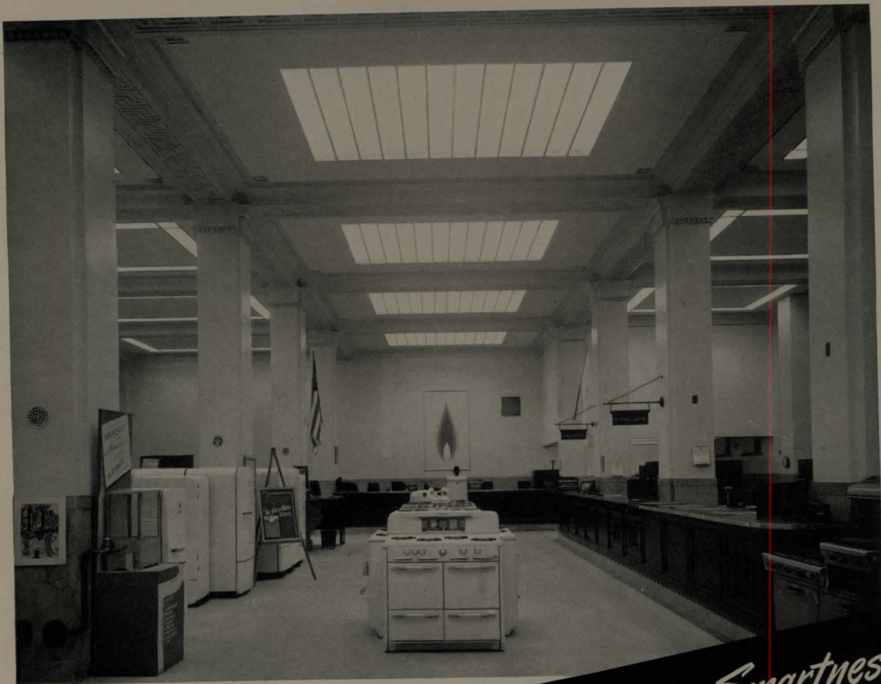
Typical Luminous Lens Ceiling installations, averaging 70, 76, and 96 Footcandles.
