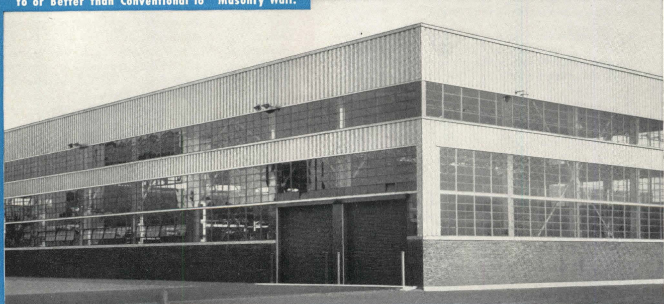
New Plant for Budd Mfg. Co. Insulated Metal Walls employed here are Mahon Field Constructed Fluted Type, with Exterior Wall Plates of Aluminum. Giffels & Vallet, Inc., L. Rossetti Archt. and Eng., S. N. Nielsen Co. Gen. Contrs.
