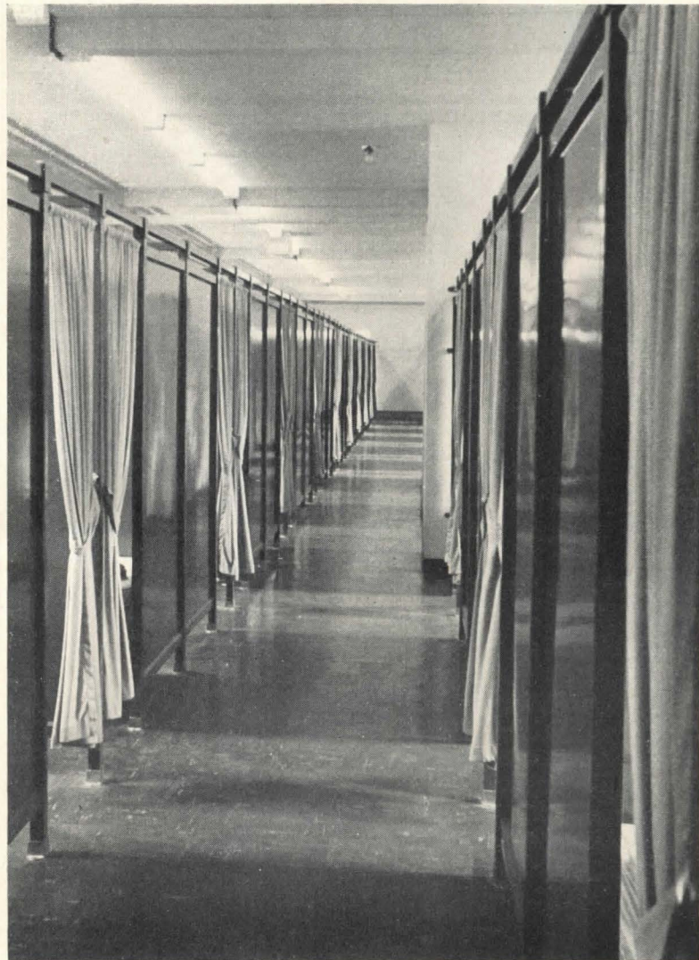
Living quarters are located on second floor (above) and in basement (below left). Dormitory cells (below) are separated by metal half-partitions, equipped with bed and wash basin. Floors throughout are asphalt, most lighting fluorescent with remote-control wiring
