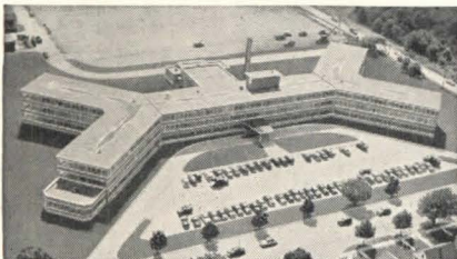
New Jersey State Highway Office Building, Trenton, N. J. Micklewright & Mountford, Trenton, Architects; Runyon and Carey, Newark, Consulting Engineers; Philip S. Slack & Co., Trenton, Heating Contractors.
