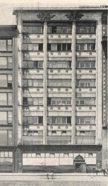
Louis Sullivan's Gage Building of 1898 . . .
