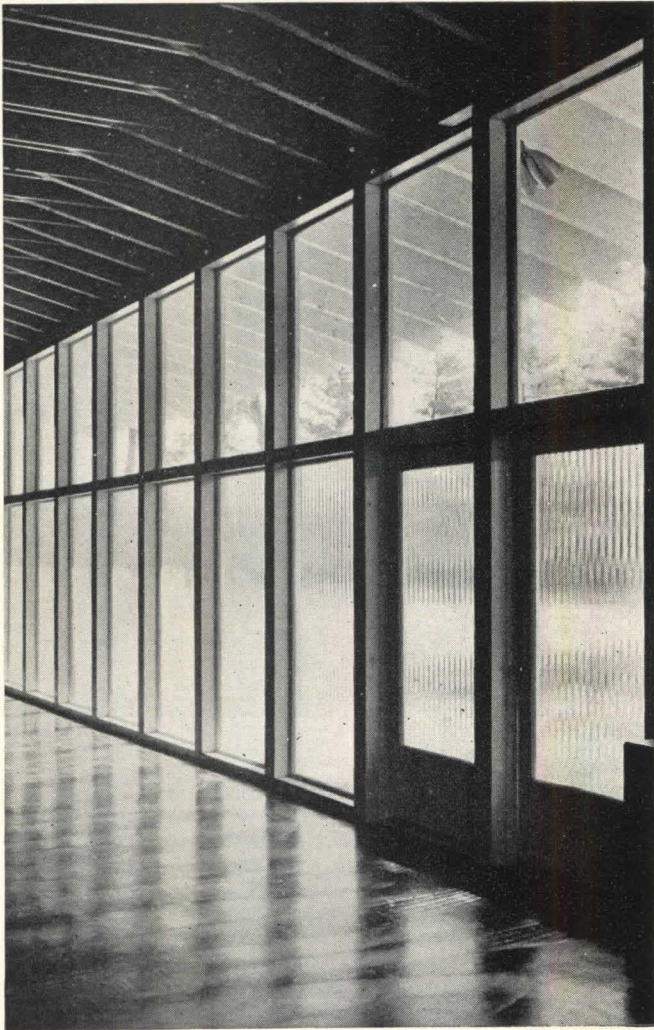
Lower window sections in the auditorium (left and above) are fitted with translucent glass to obscure view of simultaneous outside activities; clear glass upper sections give view of trees and sky. Exposed ceiling beams are painted a dark terra cotta, and extend to form sunshade over south windows. Roof is surfaced with white marble chips
