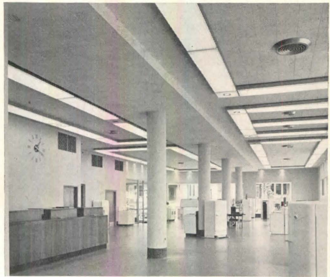
Above: private office with room air temperature controlled by the unit conditioner under the right-hand window. Ventilation air comes from duct above the windows. Piping for room conditioners of floor above is located alongside this duct. Below: first floor, temperature controlled by air supply alone
