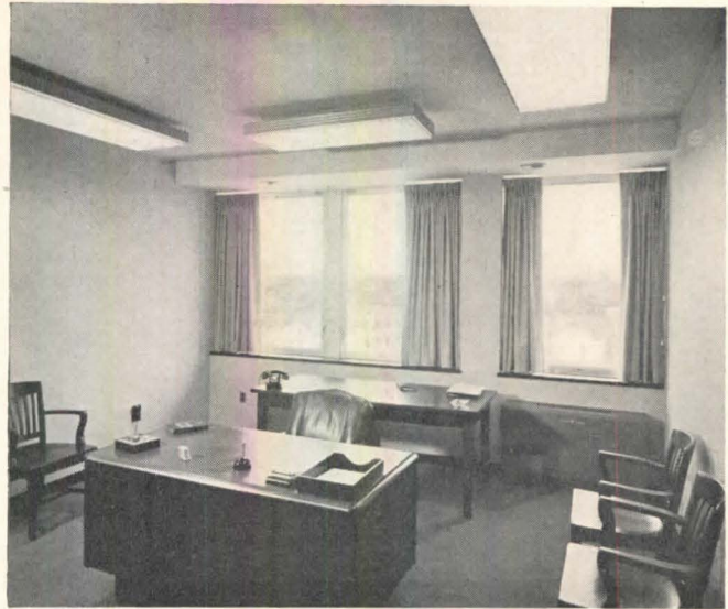
Above: private office with room air temperature controlled by the unit conditioner under the right-hand window. Ventilation air comes from duct above the windows. Piping for room conditioners of floor above is located alongside this duct. Below: first floor, temperature controlled by air supply alone
