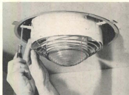
Single electric unit is heater, air circulator, light. Exterior grill not shown
