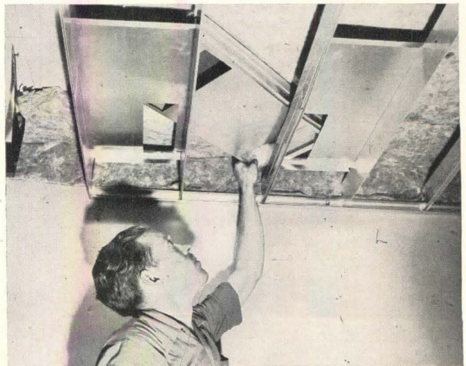
Installing the trough crossover
