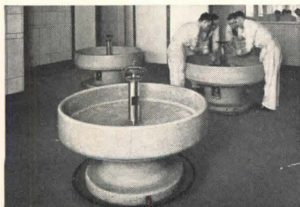
Above: Typical installation of Bradley Washfountains showing the 54" full-circle model.
