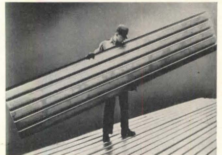
Size of new steel roof deck gives labor savings, design flexibility
