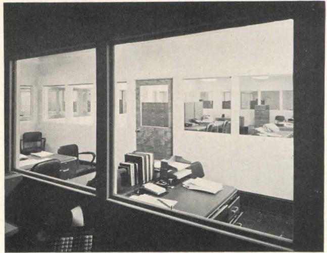
Left: conference room on second floor. The whole executive suite is paneled in Philippine Mahogany. Right: interior partitions are independent of metal tile ceilings to permit partition rearrangement
