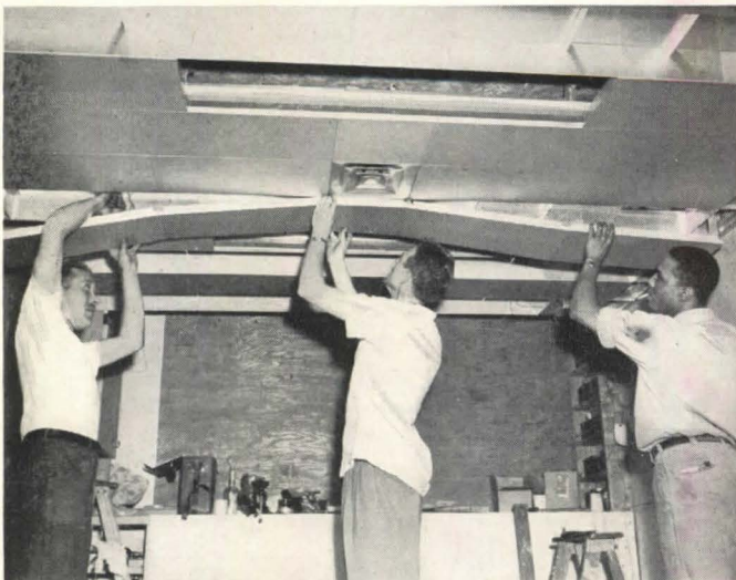
The ceiling air panel being attached
