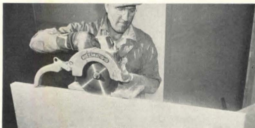
Curtain walls in Leslie R. Porter Co. office (top) are fastened by grooving laminated panel edges (above left) and inserting concealed splines (above right)
