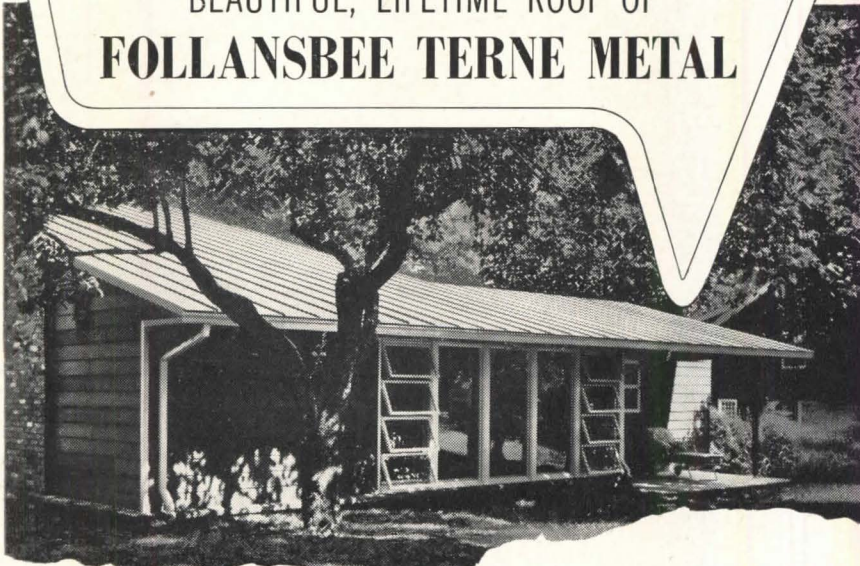
Roofing Contractor: Limbach Co., Pittsburgh, Pa.
