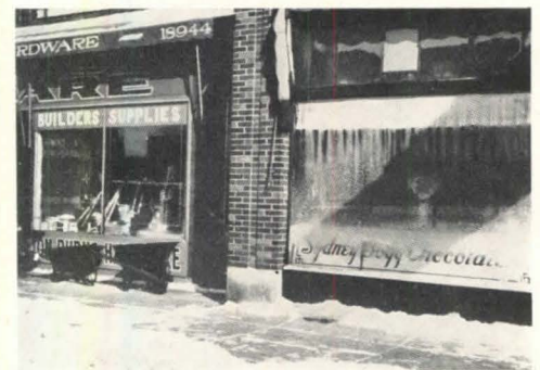
Occupancy of a building determines the amount of water vapor present. Confectioner's store, right, shows high humidity level compared to hardware store, left
