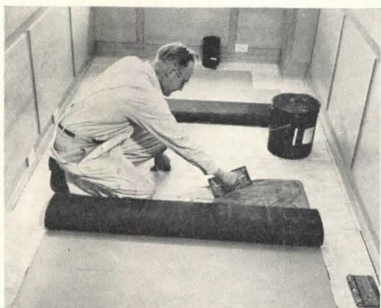
Above: striated plywood blocks form an interesting pattern for indirectly lighted ceiling. Below: fir plywood offers smooth, solid base for finish flooring. Workman is laying floor covering over \frac{3}{8} -in. stock
