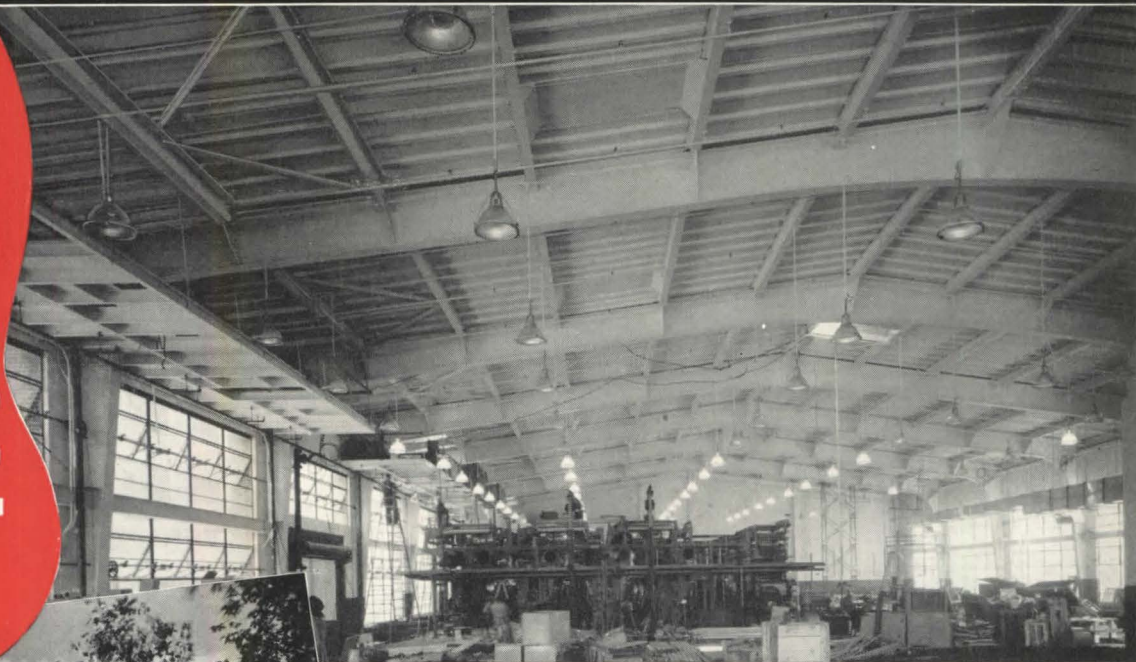
R. R. Donnelley & Sons, Co., Chicago, with over 31,000 sq. ft. of Federal-Featherweight Precast Channel Roof Slabs. Archt. Albert Kahn Associated Architects & Engineers Inc., Detroit; Contr. Peter Hamlin Constr. Co., Chicago.
