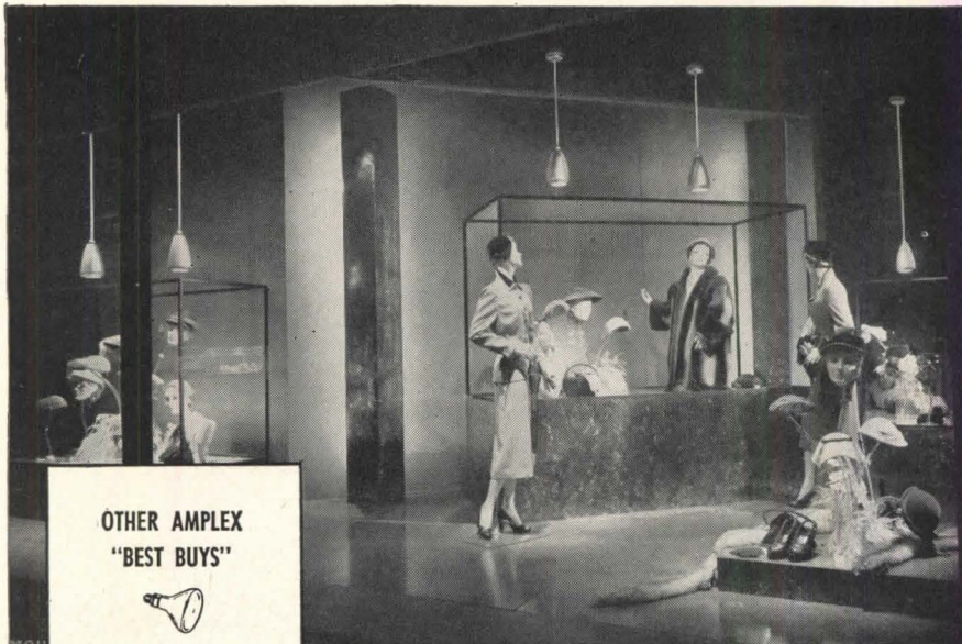
Modern accent lighting with Amplex Swivelites has brought Famous-Barr Department Store, St. Louis, Mo., top display efficiency and permanent cost savings.
