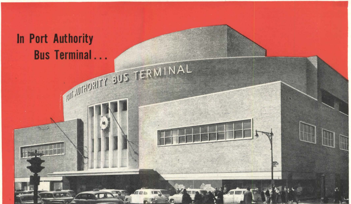
Bus Terminal Building, Port of New York Authority, Turner Construction Co.—Contractor
