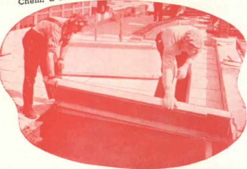
Illinois Institute of Technology, Chicago, Chemistry Bldg. & Chemical & Metallurgy Bldg., with a total of 36,500 sq. ft. of Federal-Featherweight Precast Concrete Roof Slabs., Archt. L. Mies van der Rohe, Chicago; Contr. Dahl-Stedman Co., Chicago, Assoc. Archt. Chemistry Bldg., Friedman, Alschuler & Sincere, Chicago, Assoc. Archt. Chem. & Met. Bldg. Holabird & Root & Burgee, Chicago.
