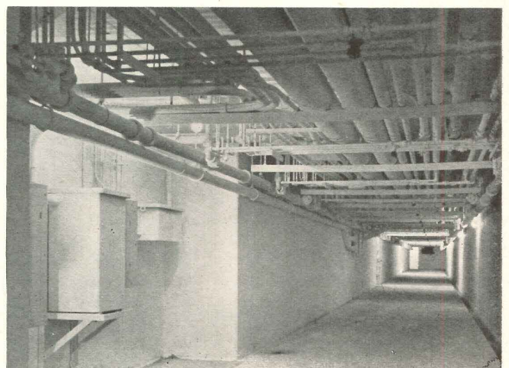
Service piping tunnels under laboratories are large enough to accommodate a maintenance truck
