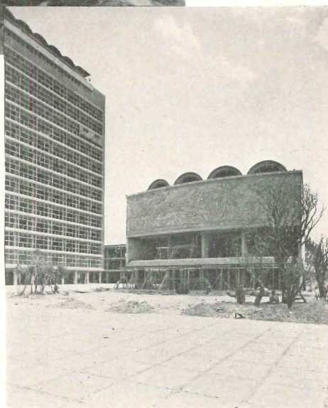
Large glass-walled building is Tower of Science, with adjoining mural-fronted auditorium. View at far right, taken from opposite side, shows science lecture halls, with auditorium at left and Tower in background
