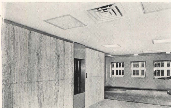
Building plan shape was calculated to give maximum number of outside offices (see fifth floor plan above center). Photos at right show mock-ups of typical offices; below, present stage of interiors
