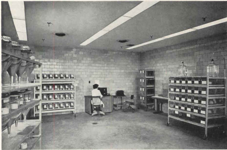
Left, animal room in laboratory wing. Below, center left, steam is supplied by three oil-fired, high-pressure boilers of a new design, each with a capacity of 24,000 lb of steam per hour at 300 lb pressure. Fuel burning efficiency exceeds 80 per cent under full automatic control. Center, right, 200-ton and 450-ton refrigeration machines; well water which has passed through air conditioner coils is reused here in condensers before being discharged. Bottom of page, chemical processing building and boiler house, seen from main plant
