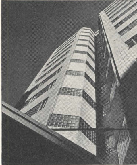
New York City's first apartment house completely planned and engineered for air conditioning by the firm of which Mr. James Mongitore is a member.
