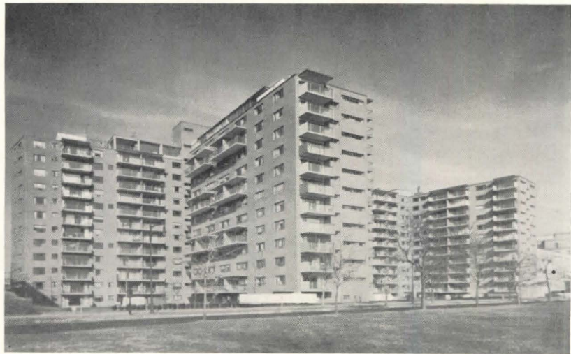
Apartment House, 100 Memorial Drive, Cambridge, Mass.; William Hoskins Brown, Vernon DeMars, Robert Woods Kennedy, Carl Koch, Ralph Rapson, Architects
