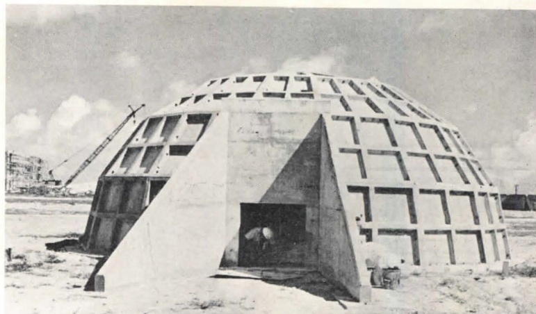
Personnel shelter designed by Navy of precast concrete
