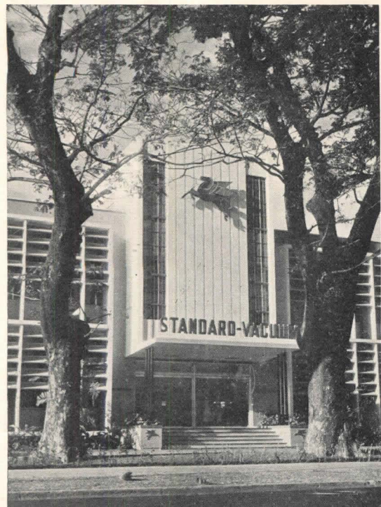
Office Building for Standard-Vacuum Oil Co. in Manila; Gonzalo Balatagas, architect. The sun control system prevents direct sunlight from entering the interior of the building at any time
