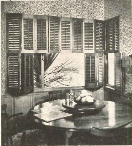
Photograph illustrated features shutters hung on a steel casement window. When installing shutters on a window of this type hanging stiles are furnished.
