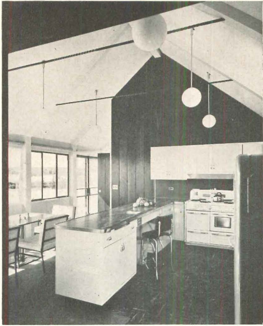
Materials were chosen to contribute to the general aspect of informality but permanence, as well as to make maintenance as painless as possible. Roof is of tile shingles; many of the floors are of slate. Heating is by radiant panel forced hot water system
