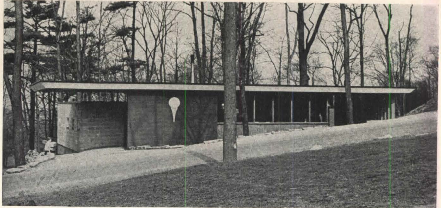
The Pro Shop for Chedoke Municipal Golf Course, at Hamilton, Ont., is built of dark brown concrete block, trimmed with light, natural wood and orange louvers; Stanley M. Roscoe, Hamilton, was the architect.
