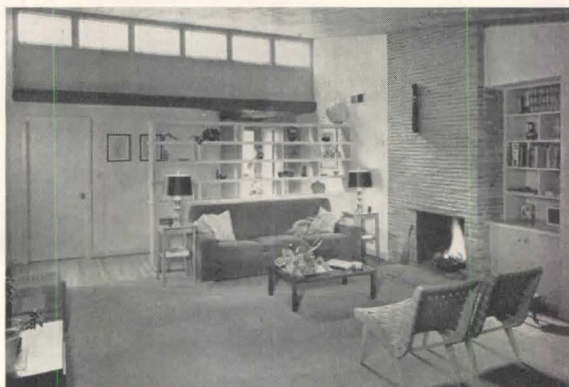
Economical square plan necessitated monitor windows for light in interior
