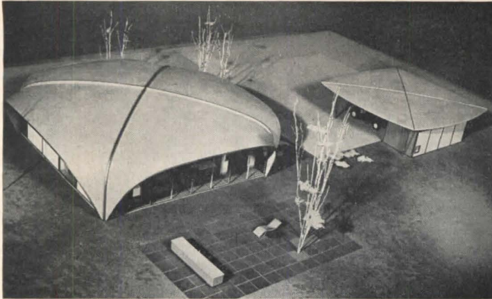
Plastic "House of 1964" designed by architect Eliot Noyes for General Electric — so far only a model for touring exhibits — has stressed-skin roof of two bonded plastic sheets, supported by aluminum ribs. Walls, partitions and floors are also of plastic. Louvered ceilings over bedrooms are made of a translucent plastic containing luminescent pigment which is electrically lighted. Circle in living room revolves
