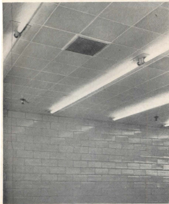
The 9-ft 3-in. ceiling, above, is finished with alternate panels of perforated metal acoustic tile or plain metal tile, with insulation between them and the roof joists to seal out dust from above. Typical office at right; the manufacturing area below
