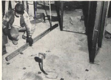
WOOD RUNNERS installed on concrete floors with MIRACLE ADHESIVE and MIRACLE ANCHOR NAILS to support 2" solid partitions. Washington Circle Apartments, Washington, D. C. GENERAL CONTRACTOR, Charles H. Tompkins Company.
