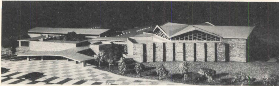
Cantilevered covered way leads to lobby from parking plaza paved in pattern of colored concrete rectangles to mark traffic lanes and parking spaces. Temple roof is formed by rigid bents tied together by central ring at valley points
