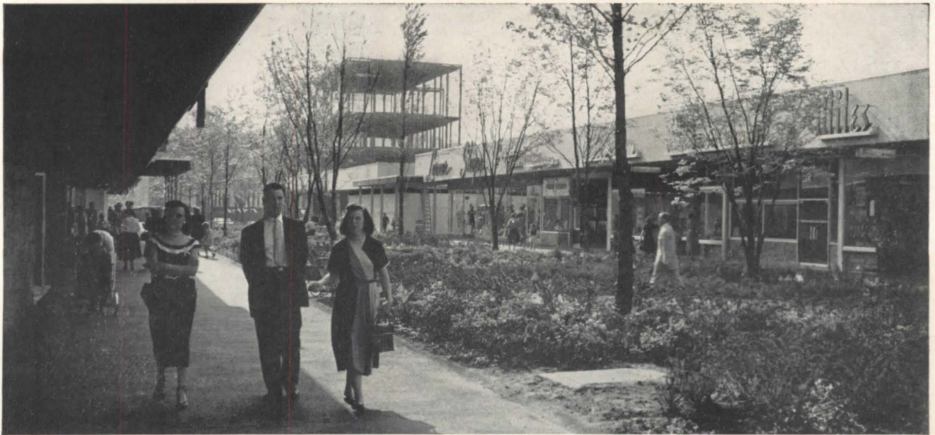
The pleasantly shaded mall, flanked by modern shops, adds charm to the Cross County Center's basically functional design. Towering in the background is the 1500-ton Bethlehem steel framework of the new Gimbel Brothers branch department store.
