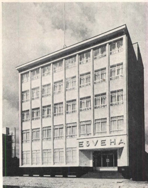
Above: J. J. P. Oud's Esveha offices, Rotterdam. Left: Lock, Amsterdam-Rhine Canal, by D. Roosenburg
