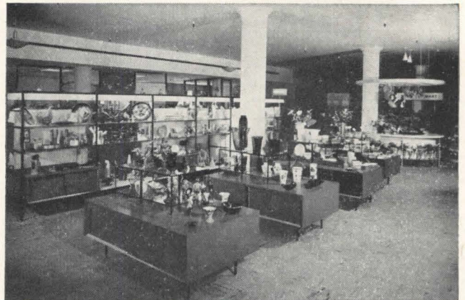
Overhead ductwork and outlets blend with the décor of Macy's—New York—gift department in their Herald Square store. Interior architecture: Copeland, Novak & Associates.
