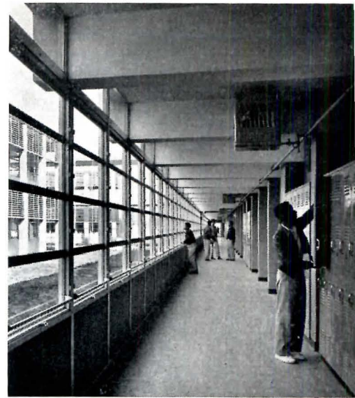
The repeated pattern of visible concrete frame, sunshades and metal louvers is evidence of the logical internal organization
