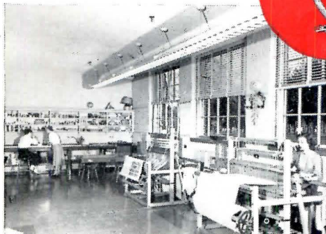
Arts and Crafts room has more than the average number of fire hazards. Here, too, Grinnell Sprinklers are constantly on guard.
