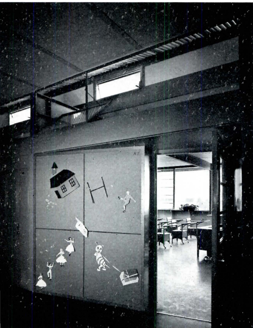
Frame is repetitive steel bents resting mostly on concrete grade beams. Floors are radiant heated concrete slabs; roofs, poured gypsum on acoustical and insulating form boards. Window walls are alternating aluminum awning sash and fixed plate glass above built-in cabinets integrated with the structure. The double-loaded corridors borrow light from actinic-glazed, ventilated skylights which light classroom interiors
