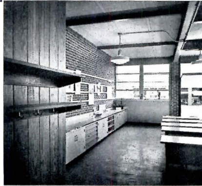
Classroom units (above and right) are all similar. Each contains 4 square classrooms, has masonry interior and exterior walls, concrete floor slab, and roof of light steel members supporting a poured gypsum deck. Program required equal and completely unified indoor and outdoor area; tilting wall is described on preceding pages
