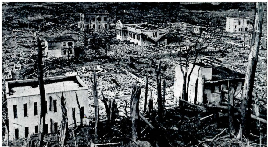
Remains of Nagasaki Medical College. Concrete buildings remaining suffered various degrees of damage from blast and fire, but others of wood were completely destroyed
