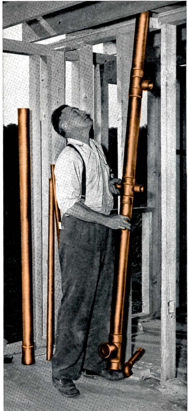
ONE MAN EASILY POSITIONS this 3" prefabricated stack which fits in a standard 4" width partition. Anaconda offers you both Type M Tube and the new lighter-weight Copper Drainage Tube, Type DWV.
