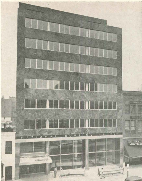
IN WASHINGTON, two more headquarters buildings opened, and another recently under way. Above left: National Housing Center, new eight-story home of the National Association of Home Builders planned as an exhibit and information center for the whole homebuilding industry; Aubinoe, Edwards and Berry,
