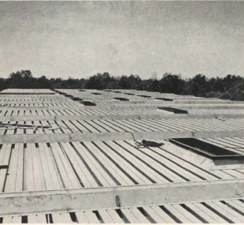
15, 16, 17, 18: Various applications, Fenestra steel roof decking; structure plus acoustical purposes
