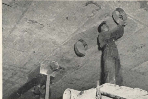
Metal gasket-straps are fastened to inserts in concrete slab
