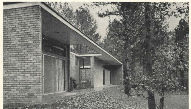
Award of Merit: Samuel T. Lemer residence, Atlanta; John A. Portman, architect, Atlanta
