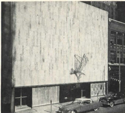
Award of Merit: Fraternal Order of Eagles Building, Atlanta; John Portman, architect, Atlanta
