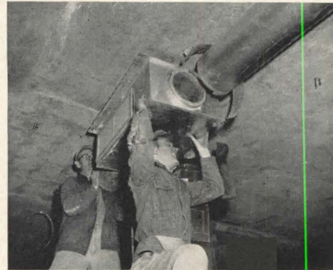
An outlet box is lifted into position
