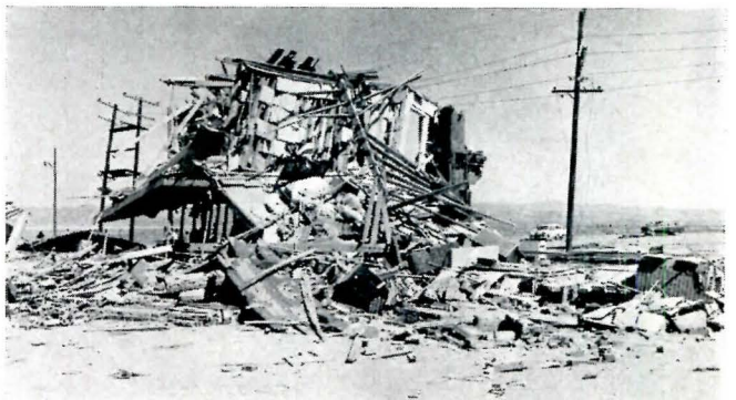
BRICK — Unreinforced two-story house; 5 psi overpressure
