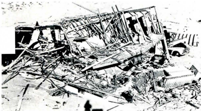
WOOD — Two-story frame house; 5 psi overpressure
