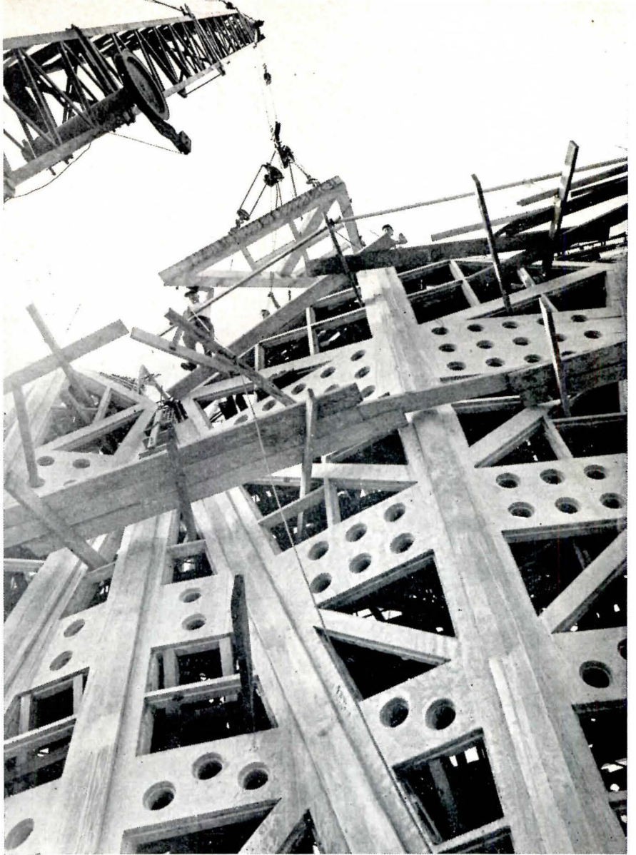
Assembly-line technique for precasting wall and roof sections for Stamford, Connecticut's First Presbyterian Church followed sequence shown at left. Forms were laid out on plywood beds, reinforcing positioned, the concrete placed and cured, and completed sections removed to allow re-use of forms. Panels were delivered to the site by truck and positioned by crane as shown above. Eight inch concrete seams join panels and foundation
