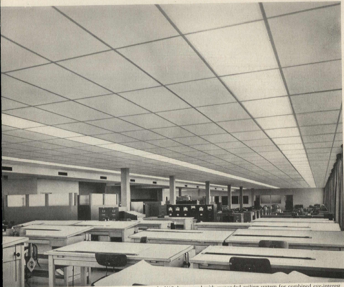
New Sylvania 2' Wide Troffers —only 5½" deep—used with suspended ceiling system for combined eye-interest and good lighting. Shown: the new offices of Hagan Chemicals & Controls, Inc., Parkway West, Pittsburgh, Pa.
