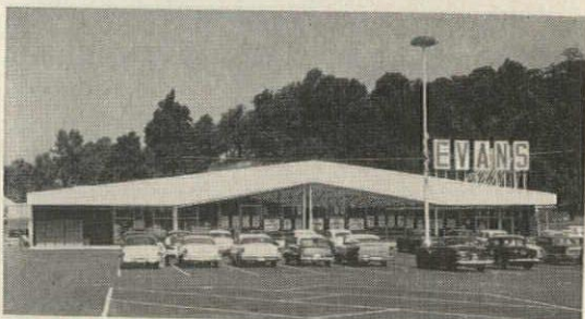
Evans Supermarket, Ashland, Kentucky. 182 x 184 foot wall bearing V-LOK frame. Erection time for steel framing — one week.
