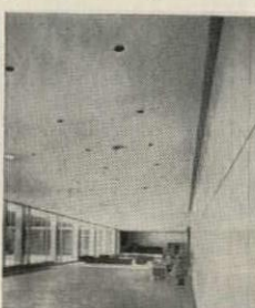
In other areas, linear diffusers, virtually unnoticeable from below, are mounted along the wall.
