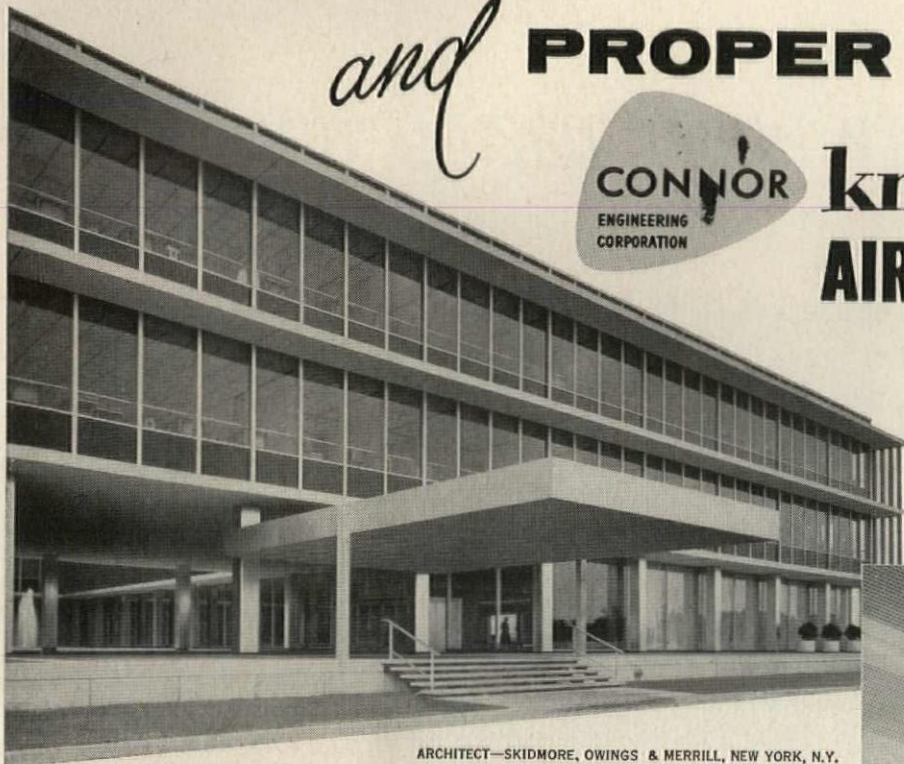
ARCHITECT—SKIDMORE, OWINGS & MERRILL, NEW YORK, N.Y. ENGINEERS—EBASCO SERVICES, INC., NEW YORK, N.Y. CONTRACTOR—HUFFMAN-WOLFE SOUTHERN CORP., CHARLOTTE, N.C.
