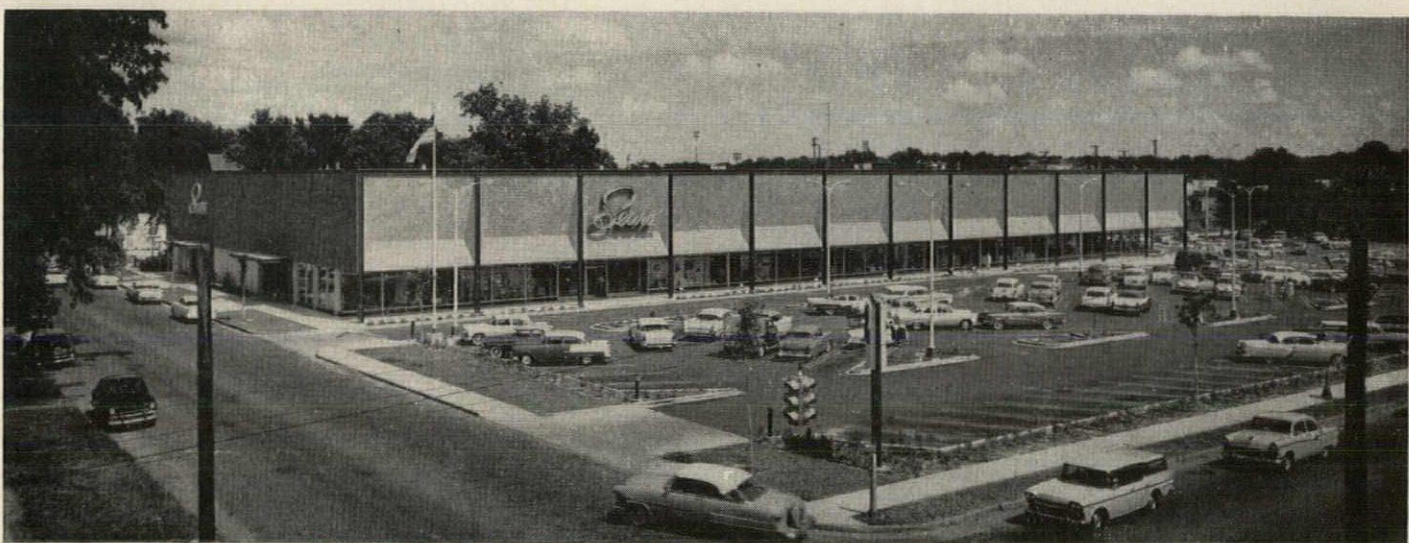
Honor Award: Retail Store, Sears Roebuck and Company, Pine Bluff, Ark.; A. L. Aydelott and Associates, Architects; Dougherty Liddell Construction Co., General Contractor
