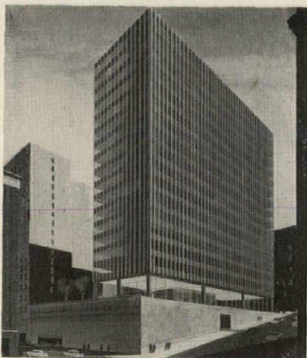
The 21-story Norton Building is to be Seattle's first major new office building in nearly 30 years. Estimated cost: more than $12 million. The plaza will feature sculptures by two Washington State men: a welded copper piece by Harold Balazs and a cast stone bird by Philip McCracken. Architects: Bindon & Wright. Consulting architects: Skidmore, Owings & Merrill. General contractor: Howard S. Wright
