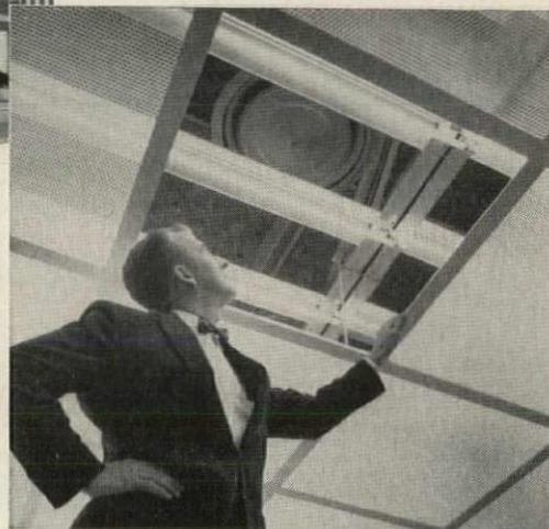
Diffuser installation above ceiling is an engineering accomplishment previously believed unworkable.
