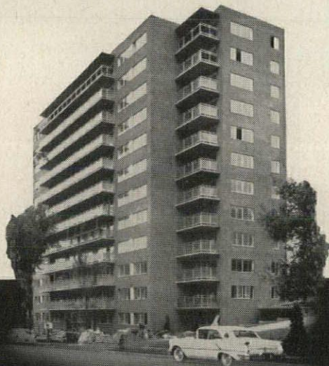
Apartment Building: Carlton Plaza, Kansas City, Missouri Architect: Herbert E. Duncan, Kansas City, Missouri Electrical Contractor: Twin City Electric Company Kansas City, Missouri
