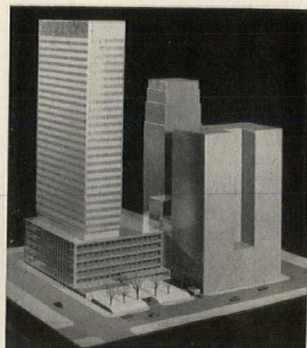
The First National Bank Building in Minneapolis is to be finished in 1960. The five-story bank portion is stainless steel, and the 23-story office tower is anodized aluminum. Underground parking and an auto-bank are below the plaza, which will be used for ice skating and seasonal displays. Architects: Holabird & Root & Burgee associated with Thorshov & Cerny. General contractor: Naugle-Leck, Inc.
