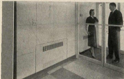
RECESSED CONVECTORS FOR HEATING
