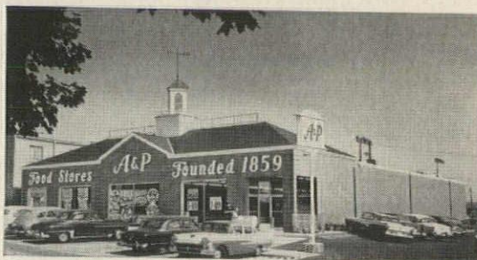
A&P Supermarket, Ashland, Kentucky. 32 x 140 foot wall bearing V-LOK frame. Erection time for steel framing only 4 days.
