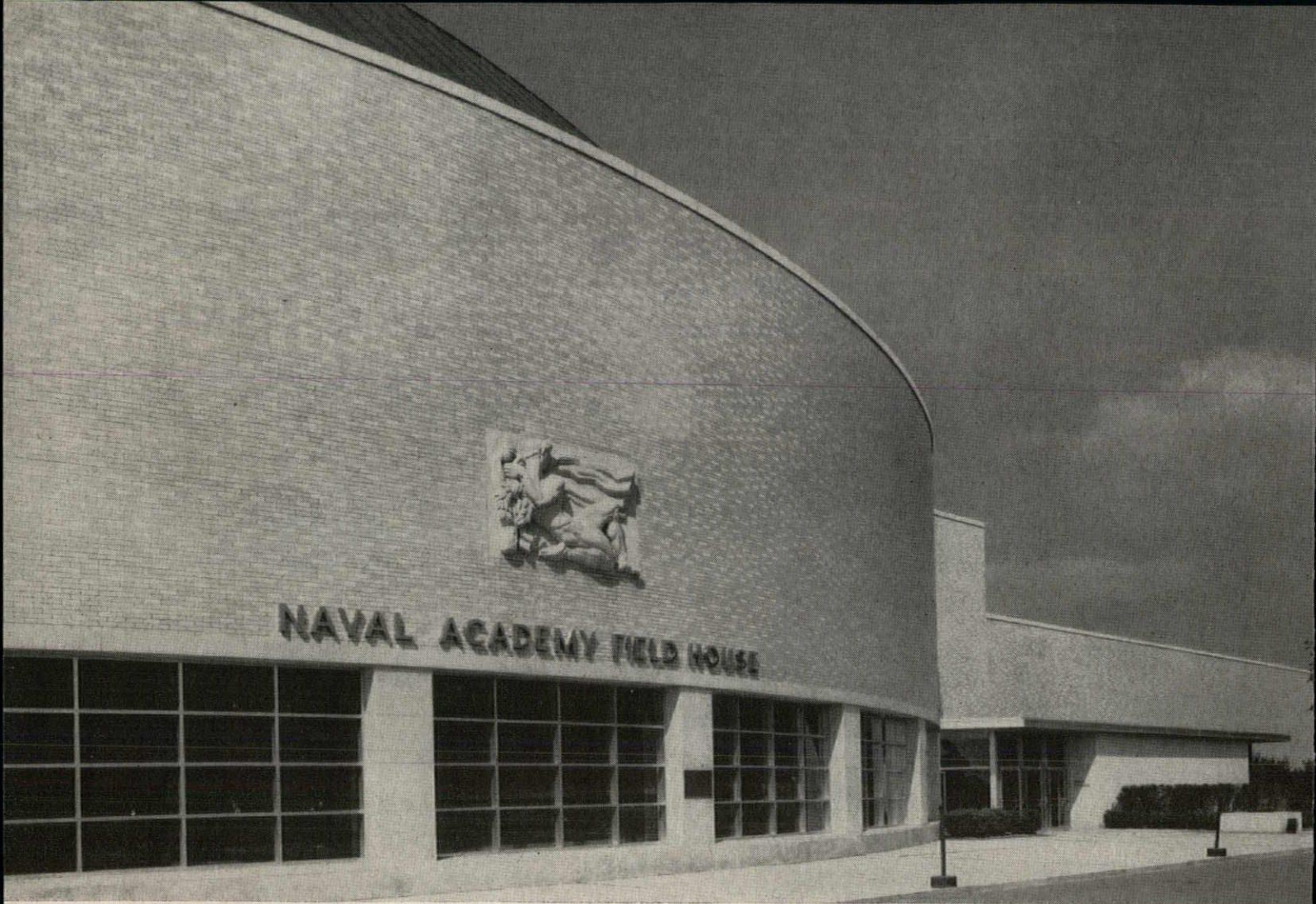
U.S. Naval Academy Field House. Architects: Harbeson, Hough, Livingston & Larson, Philadelphia, and Von Storch, Evans, & Burkavage, Philadelphia
