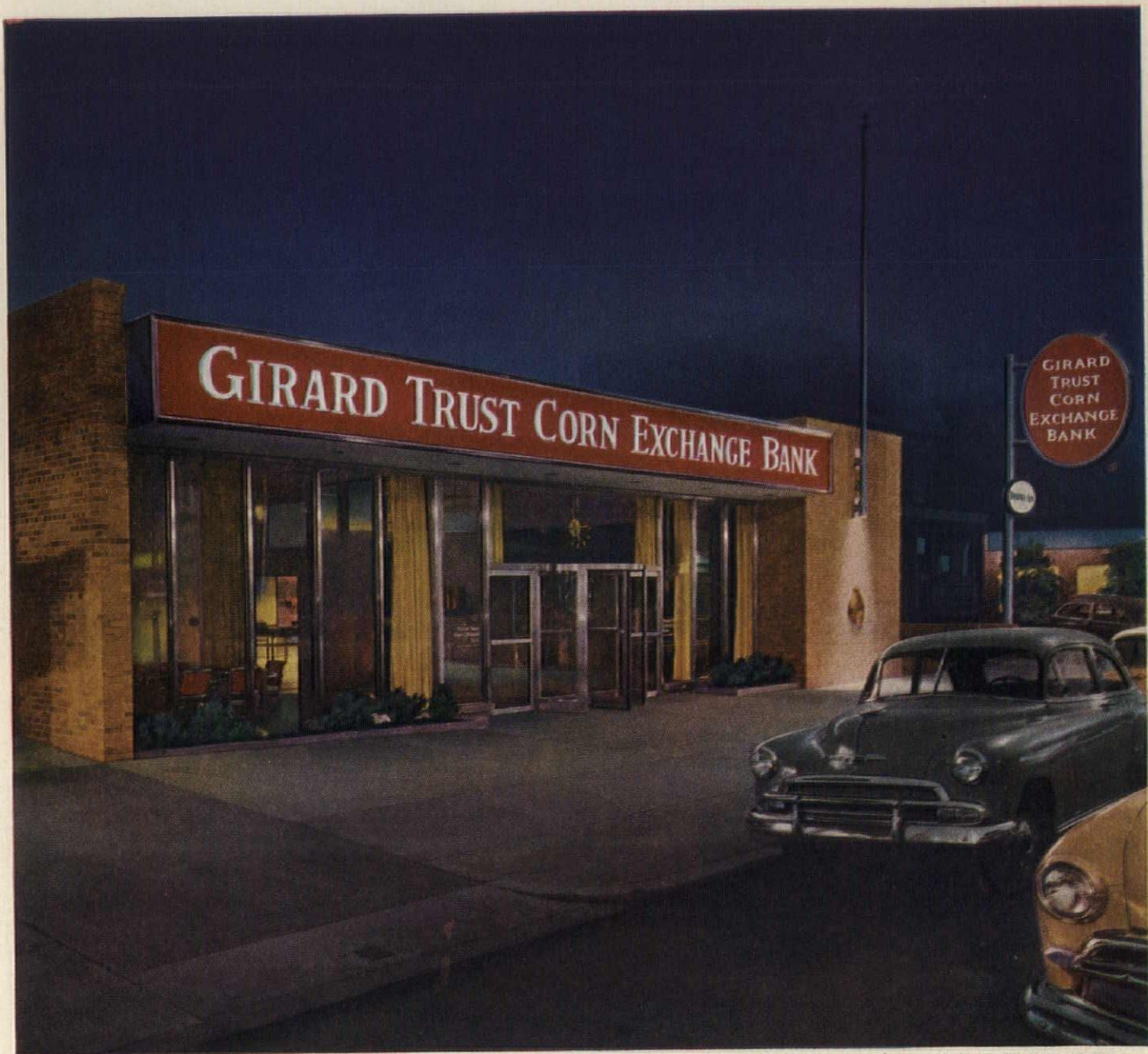
This new branch bank office in Philadelphia has completely luminous facade and oval signs with maroon PLEXIGLAS faces and white PLEXIGLAS letters. Architects: Thalheimer & Weitz.
