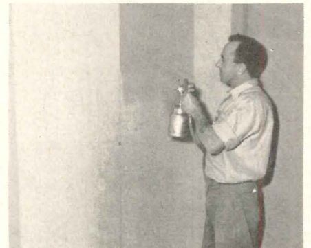
On dry wall materials like plywood, finish forms smooth protective-decorative skin
