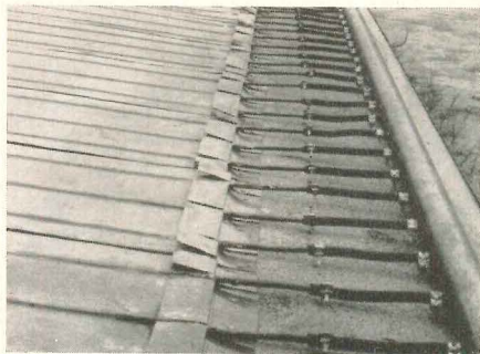
Similar panels (tubes 5 in. o.c.) are used for bare-roof type solar collector/rejector
