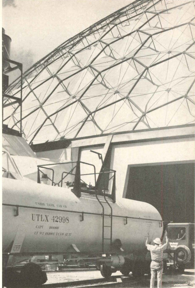
In the illustrations may be seen the usual stages involved in the handling of a tank car, from its arrival on a track outside the building, placement of the car on the rotating transfer table, and finally the transfer of the car to one of the maintenance areas
