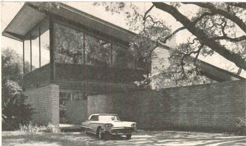
Residence in California
