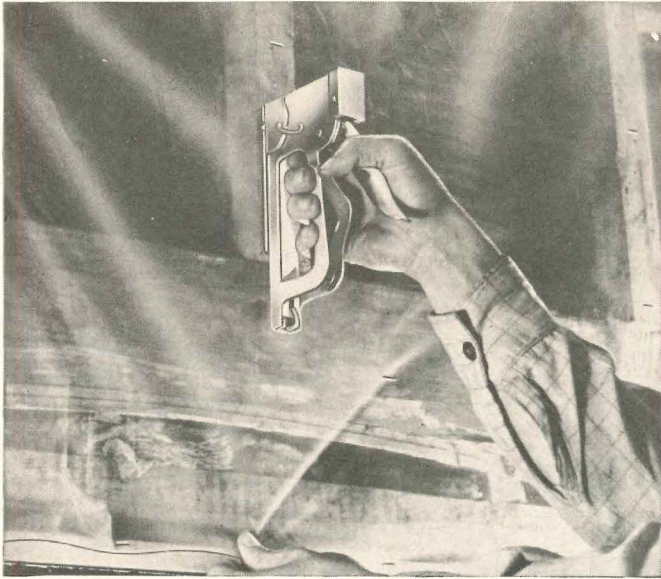
ON WARM SIDE of outside walls—VISQUEEN film protects stud walls from moisture, rot, paint peeling and checking.
