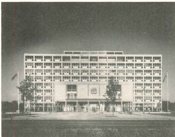
Silver Medal (category: municipal and governmental buildings): Ottawa City Hall. Architects: Rother, Bland & Trudeau, Montreal
