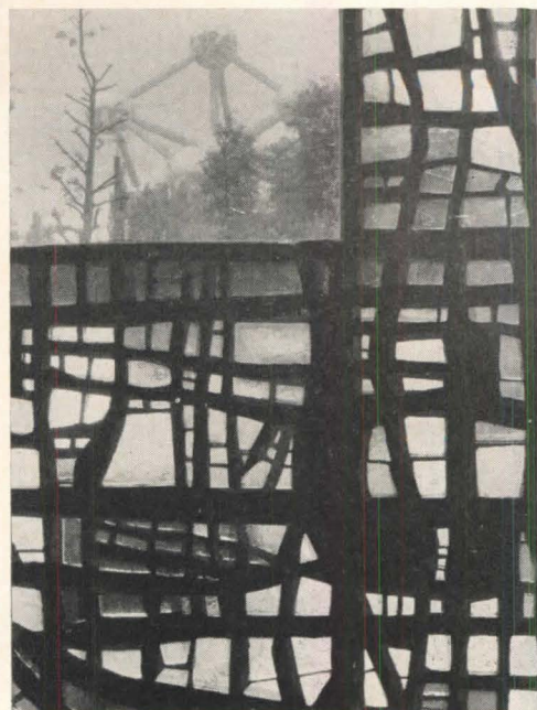
Glass-concrete panel for Dutch Pavilion at Brussels. Glass is laid in pattern on the ground; concrete poured around it
