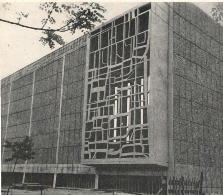
Glass-concrete window of St. Joan of Arc Church contrasts externally with exposed aggregate facings and internally with smooth, simple wall slabs
