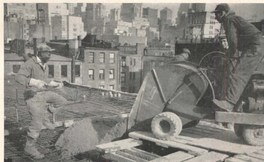
After boxes, sleeves, conduit, piping, etc. had been placed, top steel to resist negative moment over columns and spandrels was laid over 4-in. chairs and tied. Below: Construction sequence is completed by pouring light weight concrete from buggies fed by hoppers
