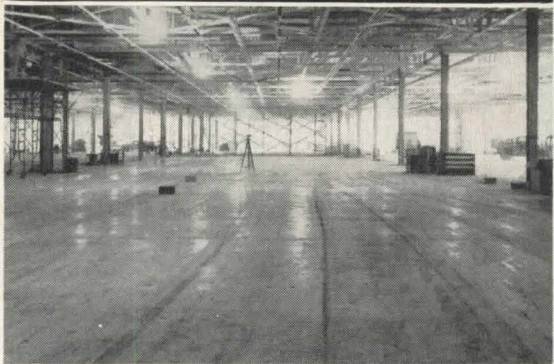
NEW CONCRETE AFTER CLEANUP
