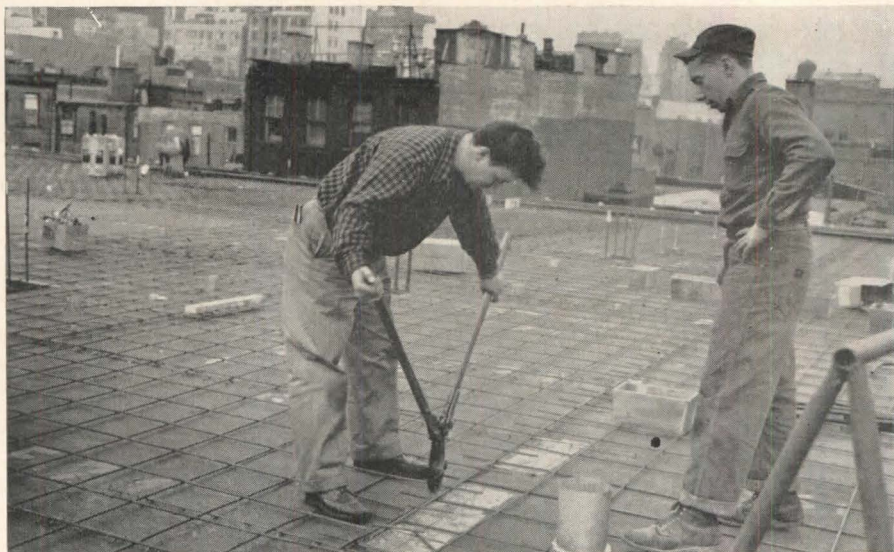
On first floor, mats were placed on top of boxes, sleeves, vents, etc. and cut away where necessary. To speed steel placement, mats on subsequent floors were laid first, as above, and cut-outs for slab breaks were later made in locations indicated by markings on forms
