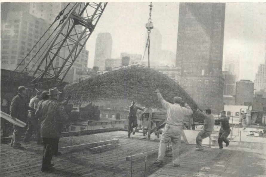
Reinforcing cage for column is lowered into form. Column and spandrel reinforcing was fabricated on the job. Below: Welded wire fabric in 19 combinations of wire spacing, gage, mat size, et cetera, is hoisted by crane, laid on previously-placed \frac{3}{4} -in. high "chairs"
