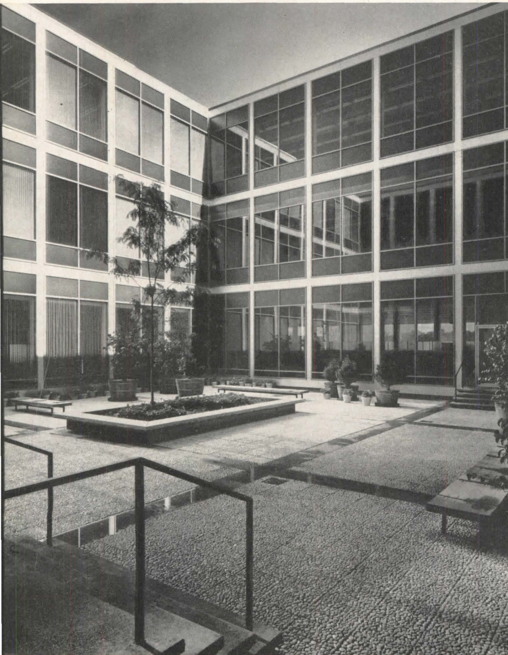
Main office area overlooks large court on first level roof. Court is completely enclosed on four sides by the aluminum and glass curtain wall, and provides additional daylight for offices
