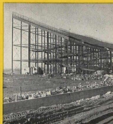
Adding new steel for increased stadium capacity
