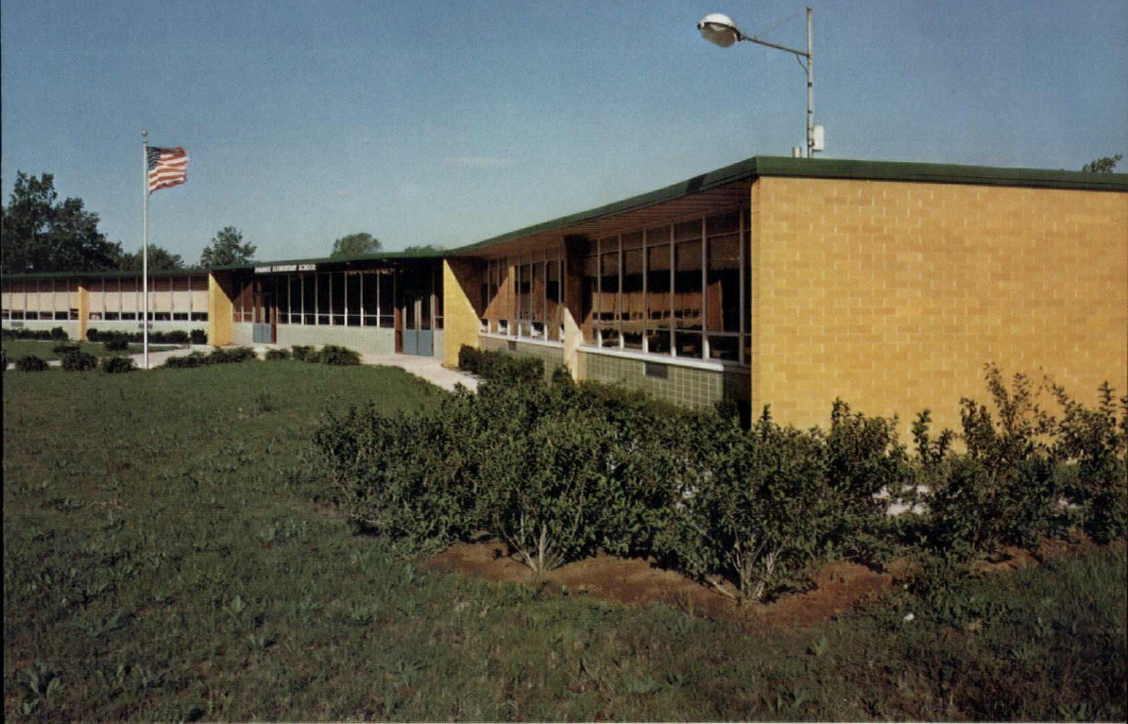
View of the modern Ivanhoe Elementary School in Gary, Indiana, showing its walls of Natco Uniwall. The buff colored vertical walls show Uniwall's exterior rugg-tex finish. The light green panels under windows show a unique use of Uniwall's interior face installed in reverse. Architect: Jos. P. Martin & Assoc.
