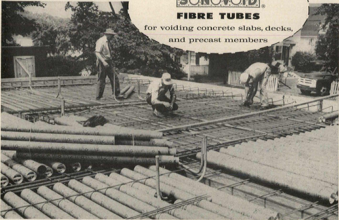
Planetarium Building, Marine Historical Association, Mystic Seaport, Mystic, Connecticut. Architect: Rogers & Butler. Contractor: A. Ceccarelli & Son
