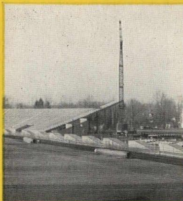
Dismantling original steel sections for removal
