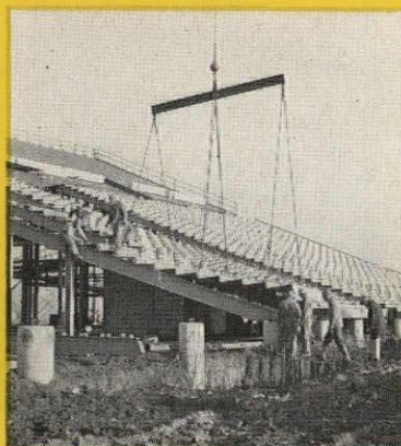
Installing original sections at new field location
