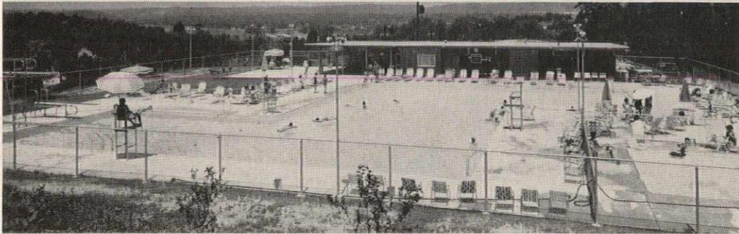
Midwest Swim Club pool by Chester, opened in Summer of 1960. "Z" shape provides two official racing courses, 25 meter and 25 yd., plus intermediate section and separate diving bay. Complete with Chester DIAVAC Filter requiring no filter room; deck-level; pre-wired, piped, and valved.
