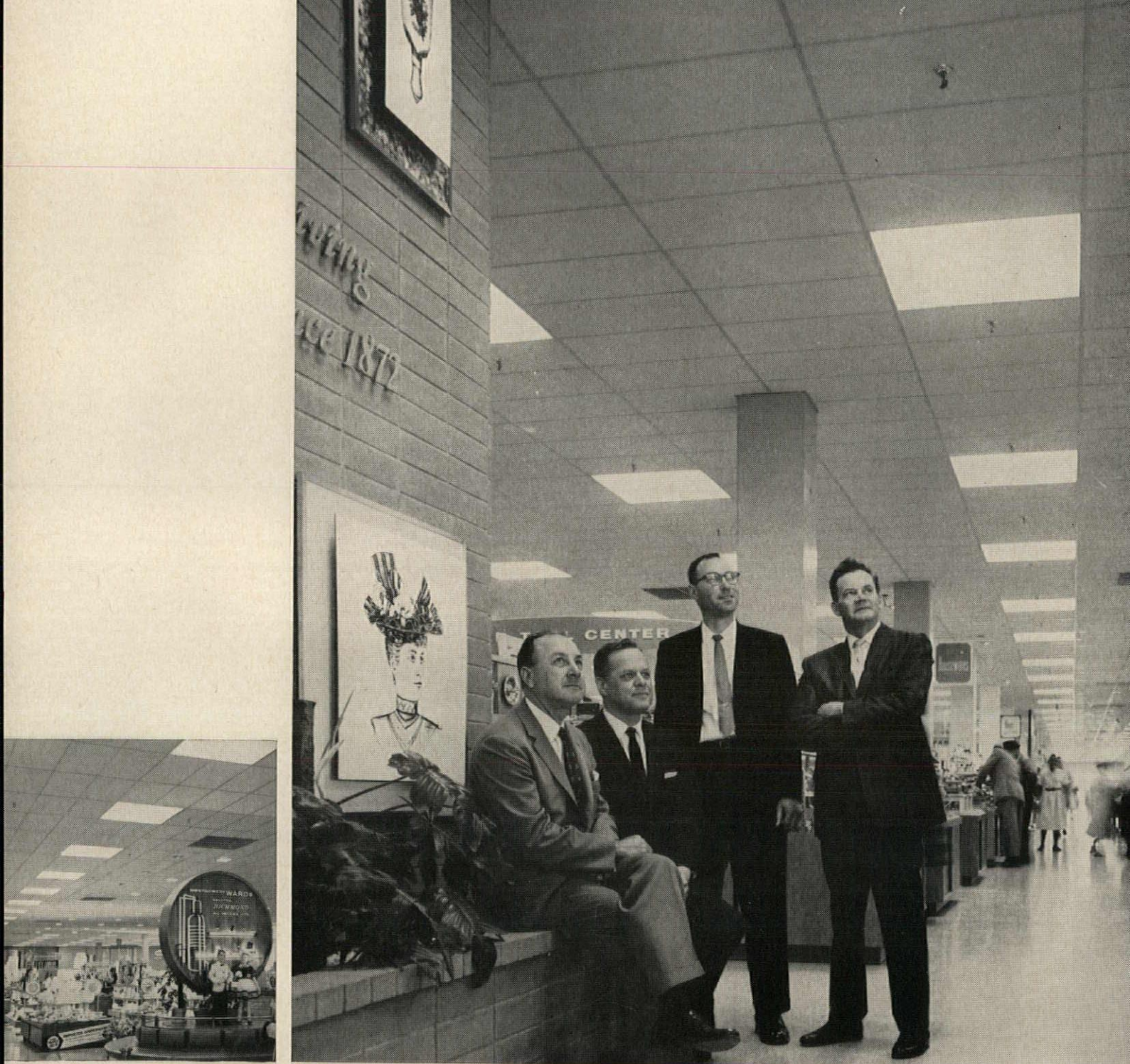
Bathing the interior with the latest in "selling" illumination are Westinghouse Mainliner fluorescent fixtures. 30° x 30° steel louver shielding diffuses the light and spreads it gently, complementing the merchandise. Ideal for large-area lighting, 700 of these handsome luminaires are used throughout the store. In photo, above, are W. K. Ostler, WESCO Branch Manager; F. L. Newlin, Ward Store Manager; C. H. Behr, Westinghouse Sales Engineer; and M. J. Muus, V. P. Newbery Electric Corp.
