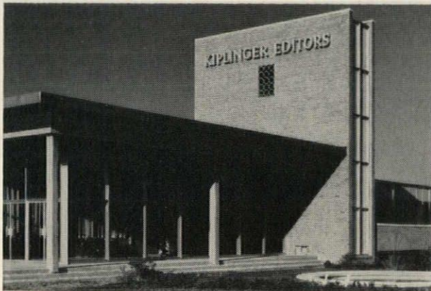
The structure of the Kiplinger Letters Building is steel frame and concrete with face brick exterior walls backed up with concrete masonry units. Built-up roofs cover the structure.
