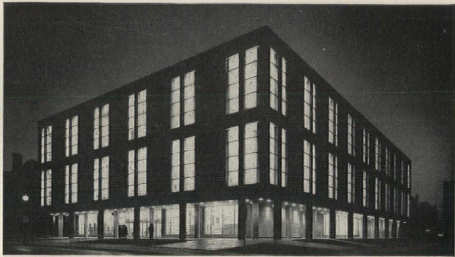
Architect and Engineer: Leo A. Daly • Electrical Contractor: Sachs Electric Corp.
