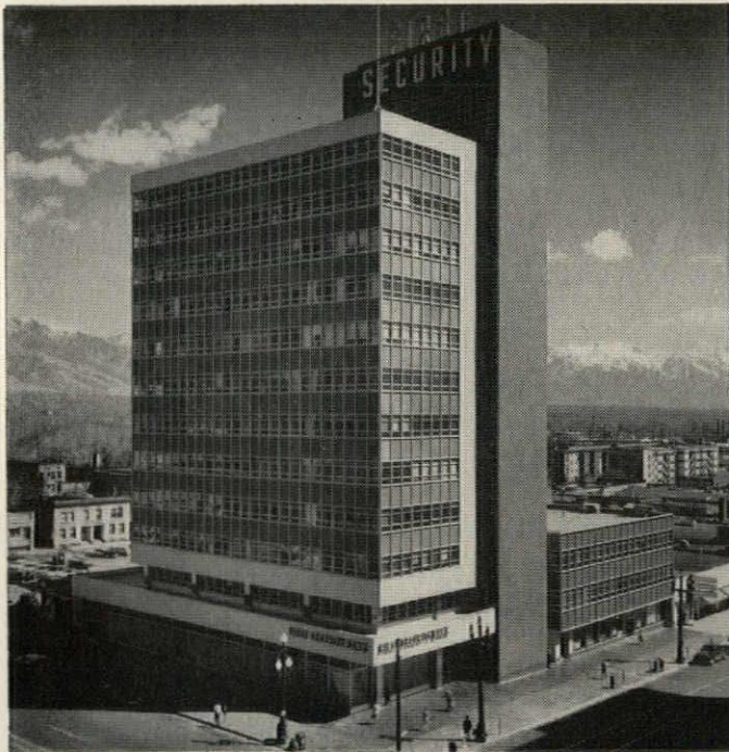
Radiant Heating and Cooling —In Salt Lake City's First Security Building, steel pipe serves a dual function. It carries steam for heating and chilled water for air conditioning. Logically, too, for steel pipe has proved efficient for heating and refrigeration, as well as icemaking, in over 70 years of service.
