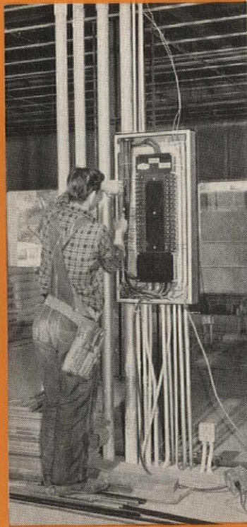
QUICKLAG CIRCUIT BREAKER PANELBOARD
