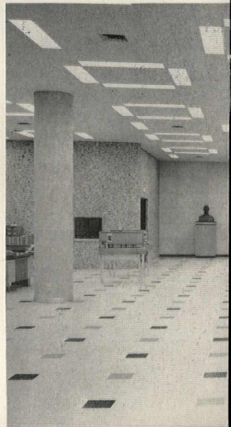
Day-Brite Troffers with Cleartex® Plastic Lens Panels deliver 73 footcandles of illumination to reading areas.
