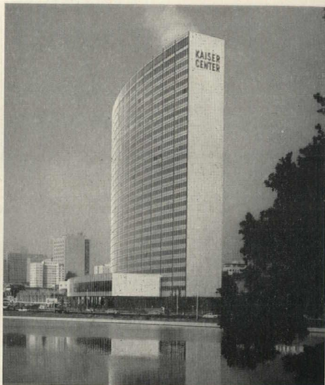
Kaiser Center—Lake Merritt, Oakland, California Architects and Engineers: Welton Becket & Associates General Contractor: Robert E. McKee General Contractors, Inc.
