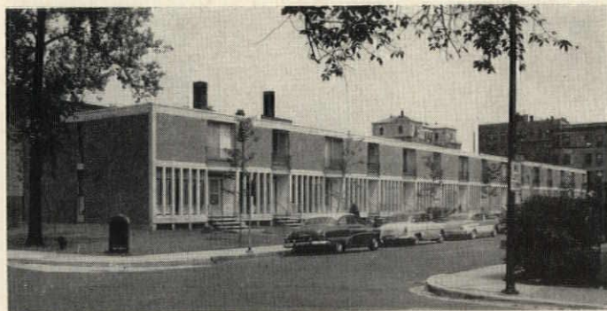
Completed Townhouses on 54th Street
