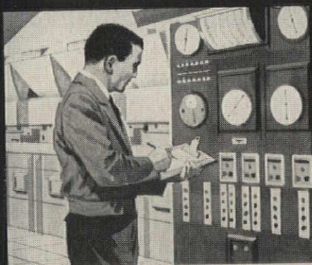
A modern boiler room in pastel colors has a clean, almost clinical appearance. Automatic sealed handling of coal and ash eliminates dust. Advance-design combustion equipment gets top BTU's from your fuel dollar.
