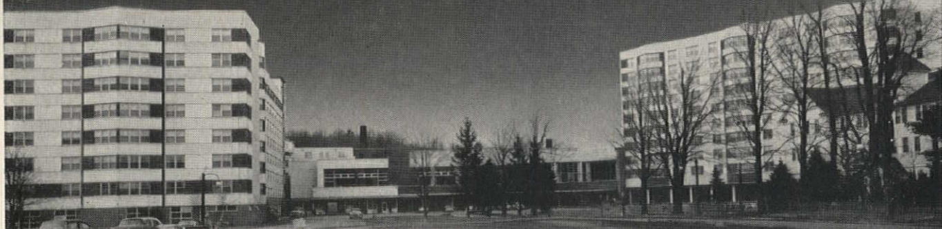
BORIS SHALMAN, Monticello, N. Y.— Electrical Contractor
