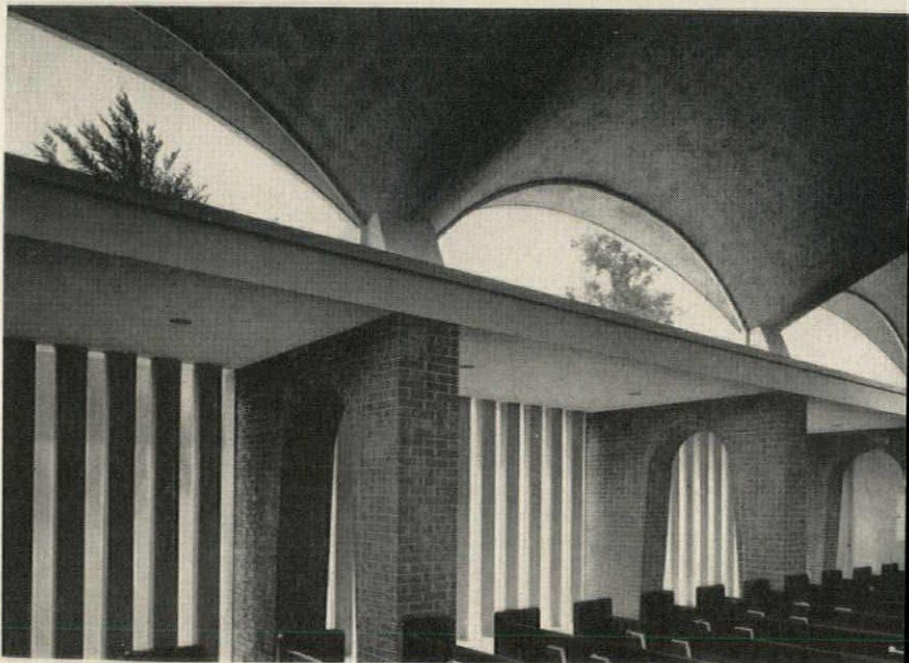
Brick veneered concrete buttresses support precast shells
