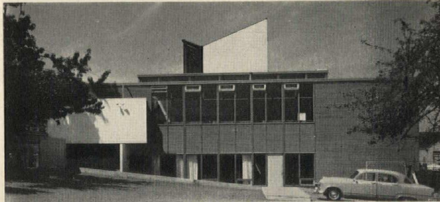
Social hall and classroom wing
