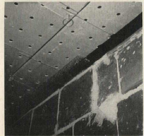
Unrestrained gypsum and metal lath ceilings with plaster casing at perimeter
