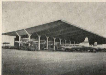
Cantilever hangar pictured at left was project No. 2 for National Airlines. Architect: Weed, Russell, Johnson and Associates, Miami; Consulting Engineer: Ammann & Whitney, New York; Soil Consultant: D. M. Burmister, New York; Contractor: Fred Howland, Inc., Miami.
