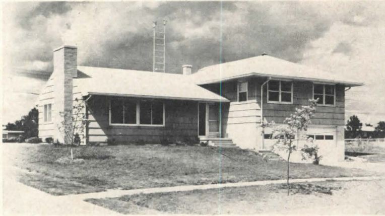
Figure 1. Warm Air Research Residence No. 4, is three-level house with concrete block walls on lower level, stud walls on upper levels
