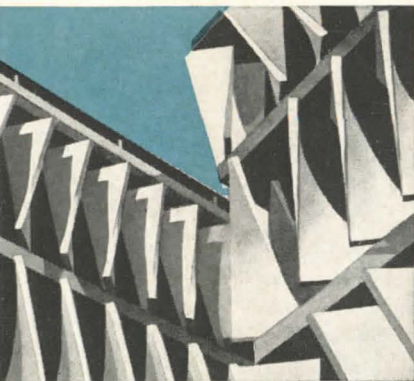
True hyperbolic paraboloids, 7'-4½" concrete panels have 90° twist, are 24" wide at top and base, 18" at waist.
