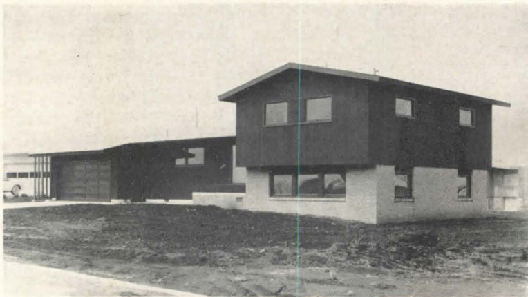
Figure 3. IBR Hydronic Research House is tri-level masonry and frame with cathedral ceilings in second and third level rooms
