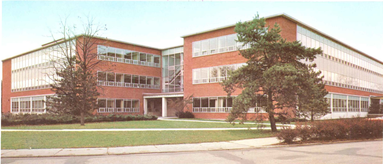
Student Services Building, completed in July, 1958, cost $18.75 per sq. ft. Windows in this building are also glazed with Thermopane for heating and (proposed) air-conditioning economies.
