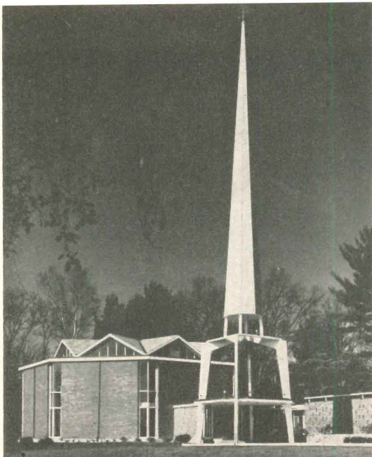
The Unitarian Church, Concord, New Hampshire. Architects: Hugh Stubbins and Associates. Owner: The Second Congregational Society (Unitarian). Contractor: A. Taylor Corporation
