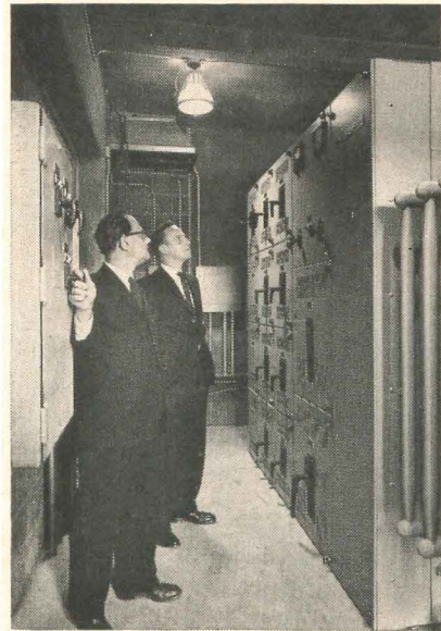
(Above) A. I. Israel operates remote circuit breaker control panel for 15 kv outdoor metal clad switchgear as R. W. MacArthur looks on. Switchgear furnishes incoming power safely and efficiently to Westinghouse 500 kva power center serving post office auxiliaries. Compact design permitted location in minimum space, freeing valuable footage for work areas.
