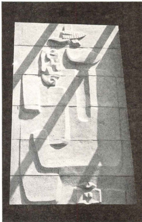
One of over two thousand 2½ ton sculptured wall panels supplied by A-M for McCormick Place, Chicago's new exhibition center.
