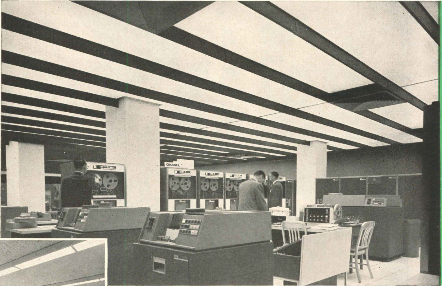
IBM DATACENTER — CHICAGO, ILLINOIS
