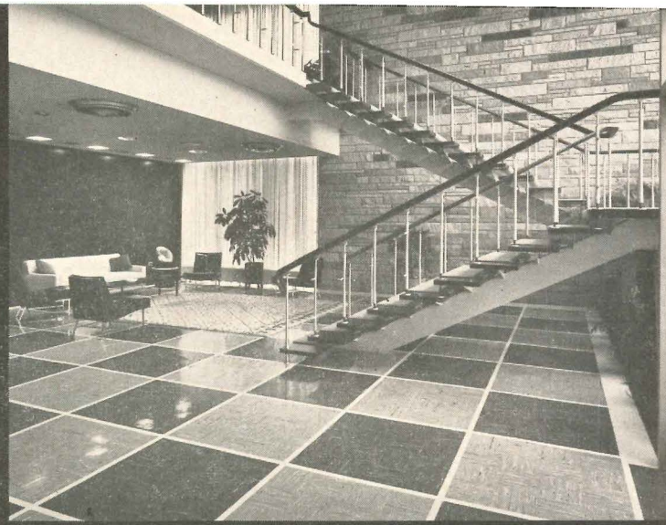
Steel-framed "floating" staircase dominates the handsome main entrance lobby.
