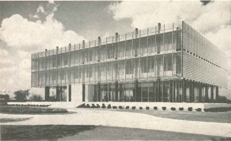
Reynolds Metals Regional Sales Office Building, Detroit, Michigan. Architect: Minoru Yamasaki. Engineers: Structural—Ammann & Whitney; Mechanical—Cass S. Wadowski; Electrical—Henry J. Guthard. Landscape Architect: Eichstedt-Johnson Associates. Owner: Reynolds Metals Company. Contractor: Darin & Armstrong Company
