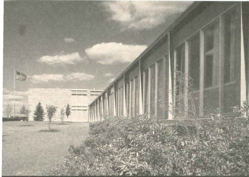
Colorful curtain walls make an eye-appealing exterior. Porcelain-enameled steel panels are blue, steel columns and beams are red.
