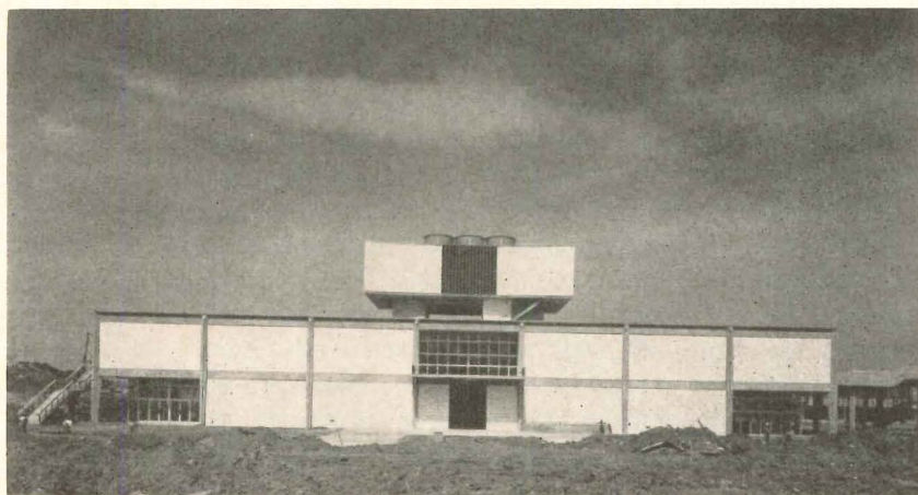
Hall Number Three, International Trade Center, Tokyo; Masachiko Murata, architect
