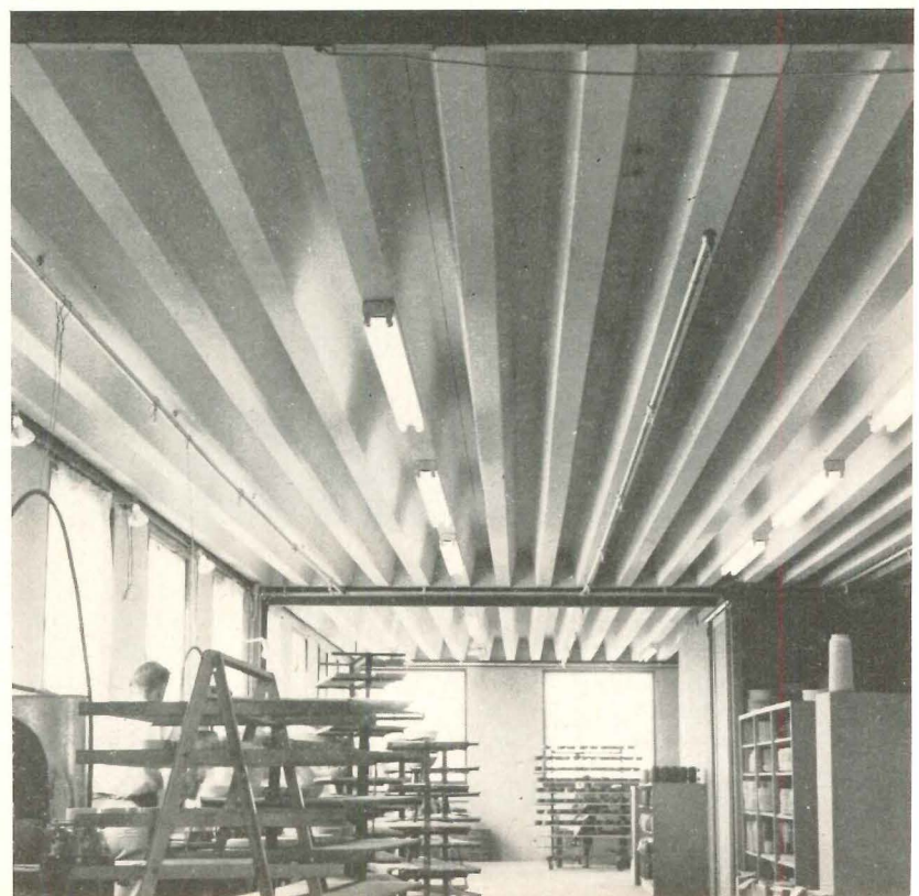
Trofdek , a miniature version of the folded plate, consists of thin sheets of plywood glued to light lumber stiffeners to form a series of troughs. The resulting roof or floor component is extremely light weight but capable of carrying loads of from 10 to 20 times its own weight over clear spans up to 50 ft. At right, it serves as structural roof and finished ceiling. Heath Ceramics Company warehouse, Sausalito, California
