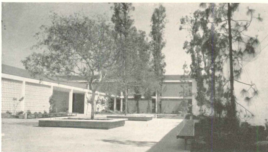
Mall between service building and laboratory, right, looking toward engineering building. Ornamental concrete grilles, left, and slat shading, center, shield covered walkways reducing heat load and providing shaded passage between buildings
