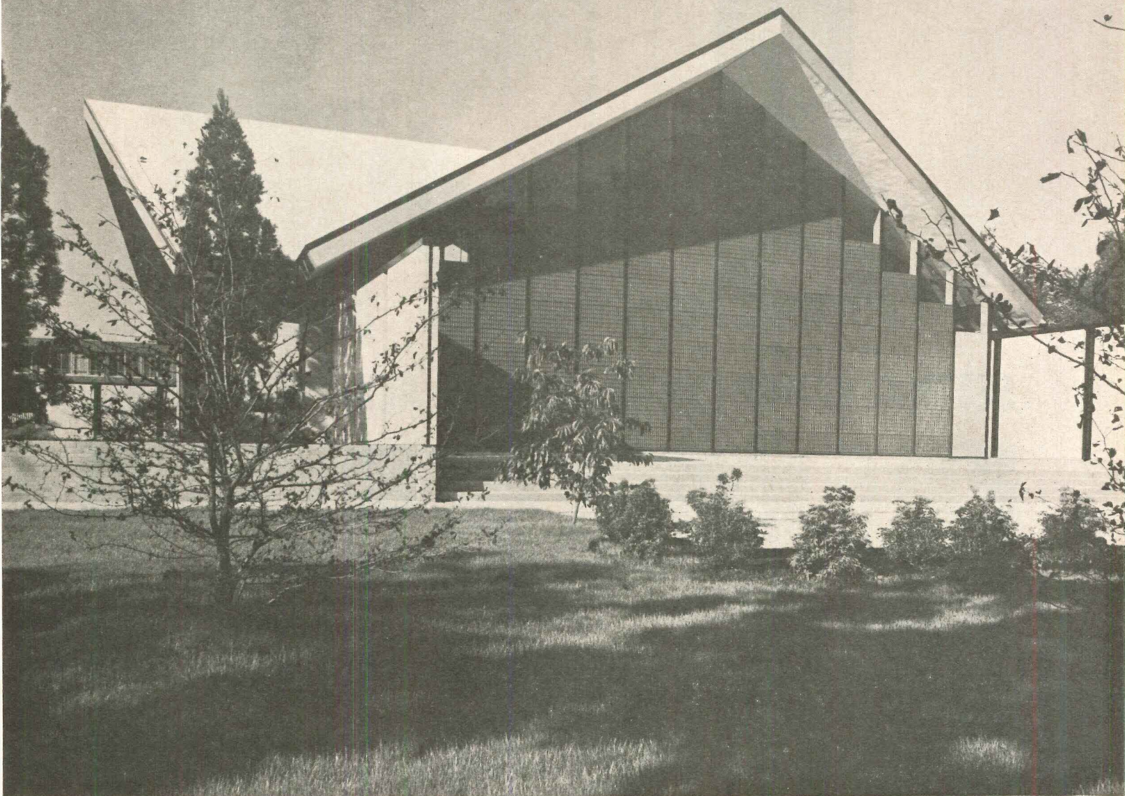
Davis, Brody, and Wisniewski, Architects
