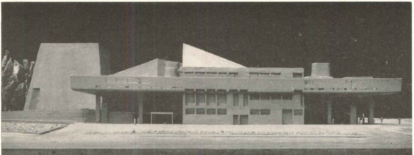
Memorial Hall, Tokyo; Kunio Mayekawa, architect
