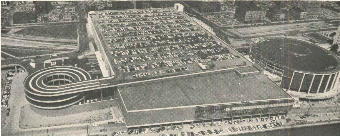
Cobo Hall covers 10 acres in Detroit's new civic center. It is the world's largest exhibition hall. One area has about 300,000 square feet of exhibit space. National Tube supplied pipe used for air conditioning, plumbing, and sewerage.
