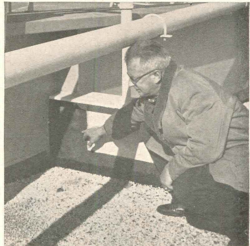
Saraloy accomplishes difficult flashing of bolted girder-purlin intersection
