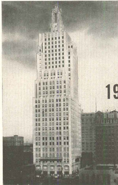
KANSAS CITY POWER AND LIGHT COMPANY, KANSAS CITY, MISSOURI
