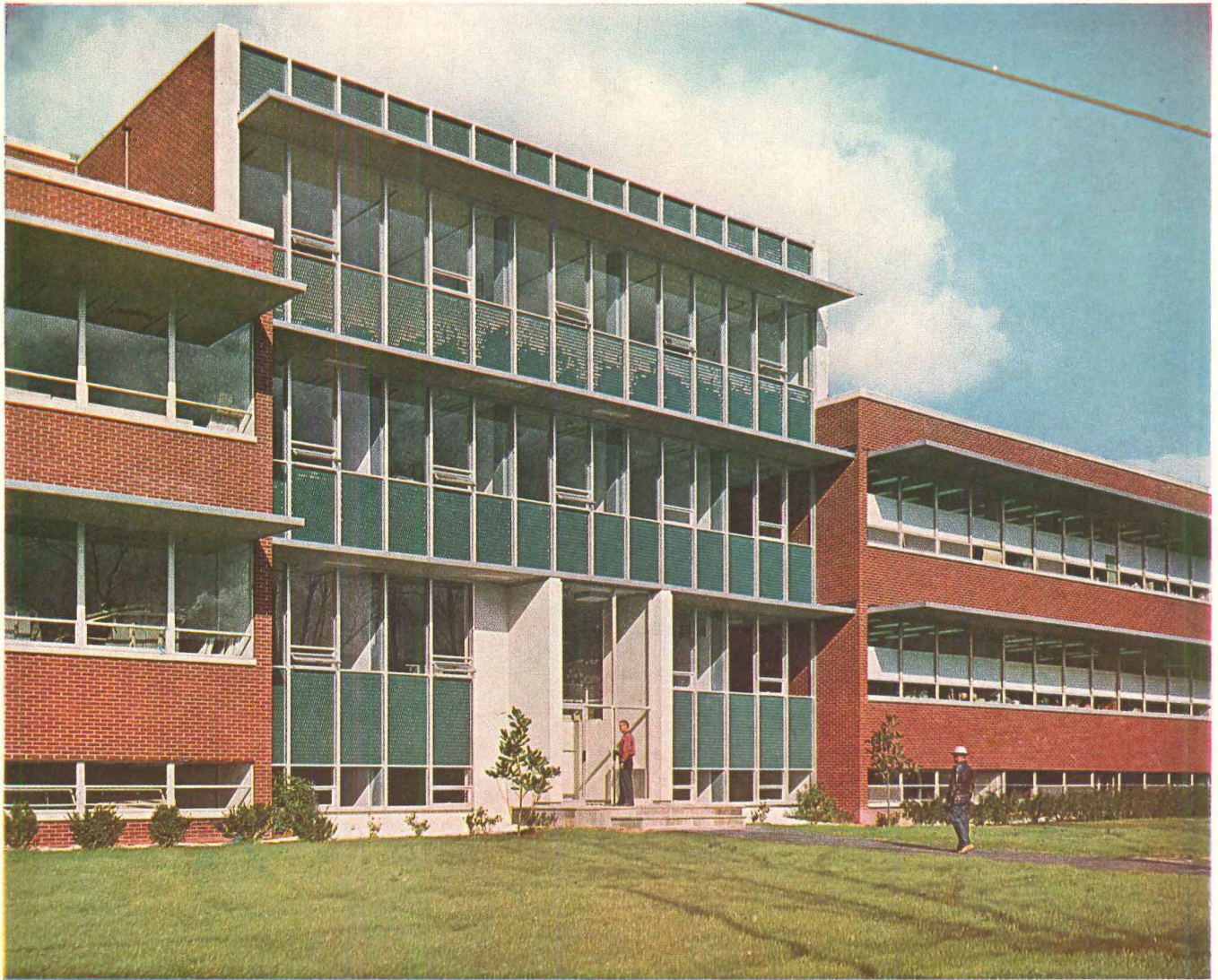
Spandrel panels of textured green PLEXIGLAS at Research and Engineering Building, Rohm & Haas Company plant, Bristol, Pa.
