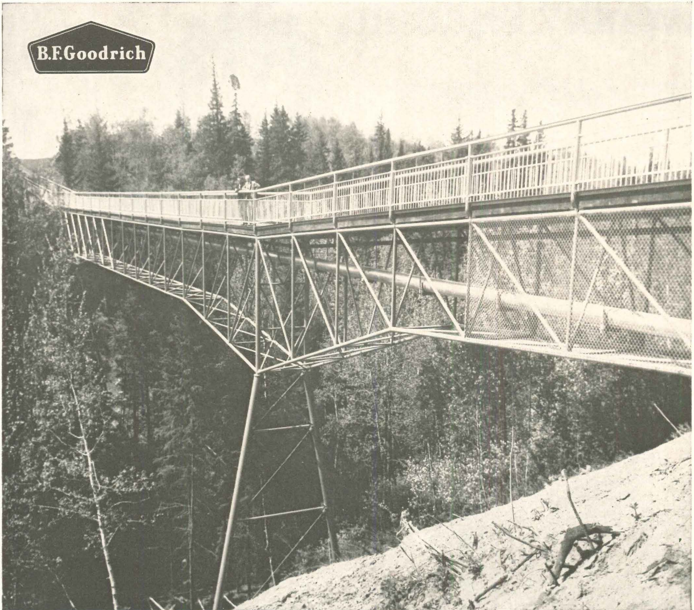
This 10" pipe of Geon is extruded by Scepter Manufacturing Company, Ltd., Toronto. Because of low temperatures, it is insulated with Fiberglas and a thin coat of aluminum. It has operated successfully through winter temperatures as low as -30^{\circ}\text{F} . B.F. Goodrich Chemical Company supplies the rigid Geon vinyl.
