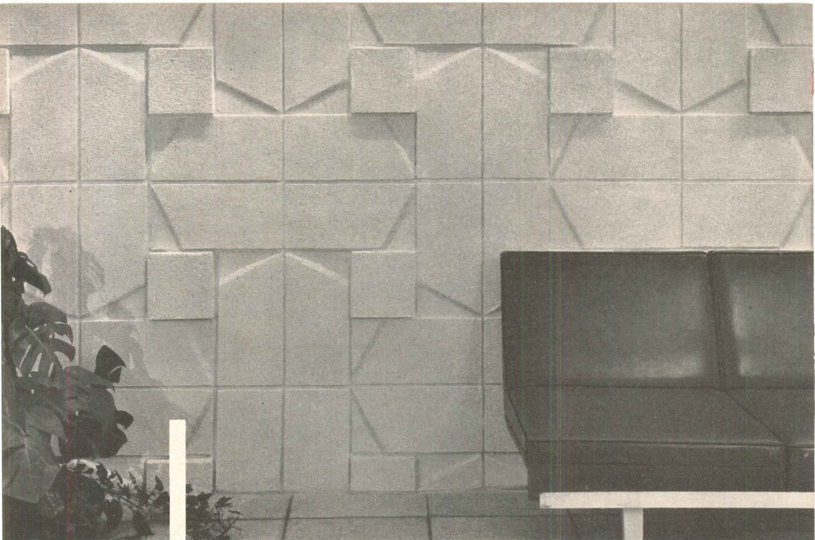
Architect Mario J. Ciampi of San Francisco blended square units with Shadowal block to form this handsome sculptured wall.
