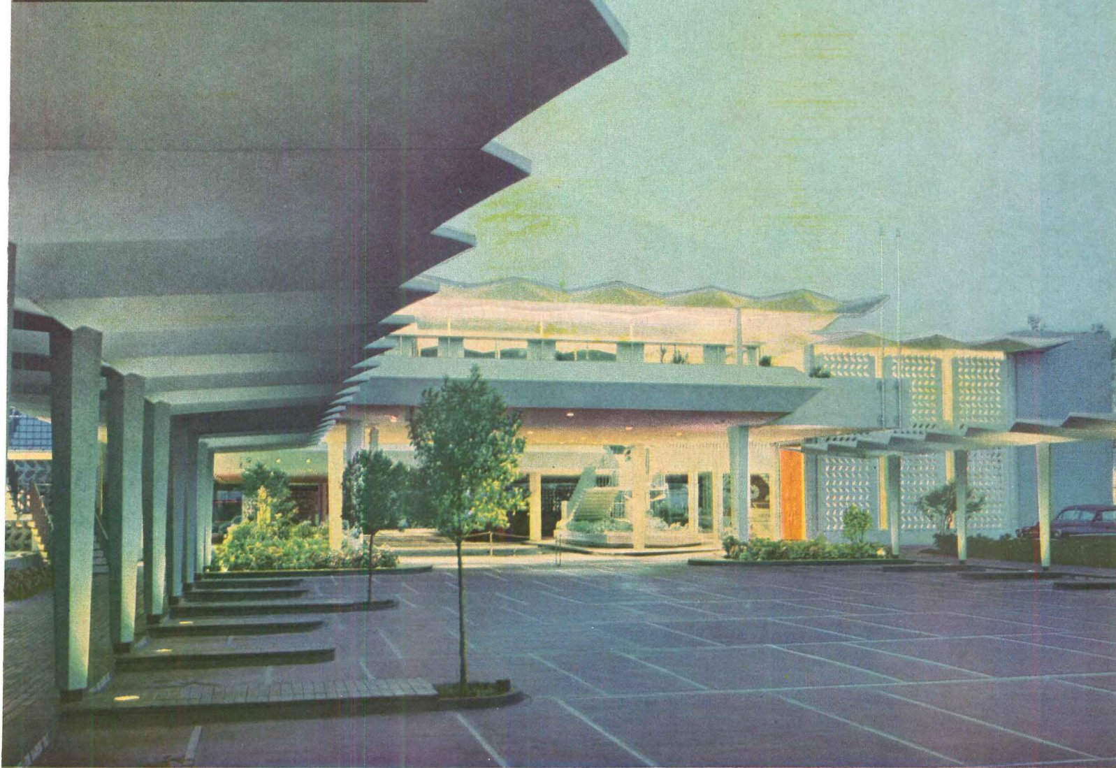
First National Autobank, Tulsa, Oklahoma. Architects & Engineers: McCune, McCune & Associates. Contractor: Tulsa Rig, Reel & Manufacturing Company, Tulsa.
