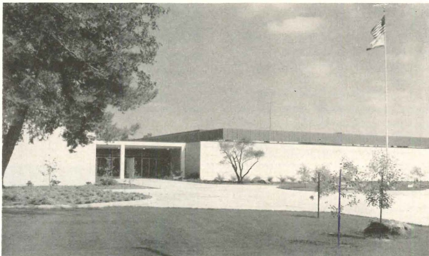
Lobby entrance joins engineering building, left, with service building. Exterior block walls are natural desert tan. Windows, used only as a design element in this project, have sea blue porcelain panels at top and bottom. Roof-mounted equipment is screened from ground view by dark brown fluted metal decking
