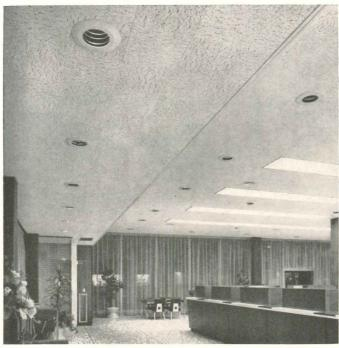
Fissured acoustical tiles for the ceiling in the Endicott Trust Building have a series of tiny holes for air supply
