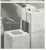
flexibility—the two basic factors for a repair-free masonry wall are assured by these engineered companion products. Dur-o-wal reinforcement, top left, increases the horizontal flexural strength of 8" concrete block walls from 60 to 135 per cent, depending on the weight and spacing of Dur-o-wal used, and type of mortar. The ready-made Rapid Control Joint, beneath, with its neoprene compound flange, flexes with the wall, keeps itself sealed tight.
