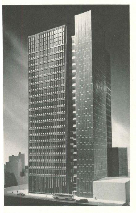
manence to the facing material, and the cost of this selection was kept in line by taking advantage of precast panel technology. A dark shade was chosen for low maintenance in Detroit's atmosphere and for contrast with other buildings at the city's hub. Its polished surface will reflect light in an ever changing expression.
