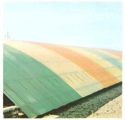
Arched panels are easily secured by cable tie-down method.
