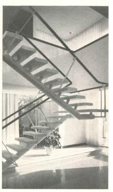
This spiral steel staircase connects three levels in a hillside home. It is composed of two strips of 3/8-inch plate, 8 inches wide. Steps are 11-gage plate with edges bent upward to form a low box to hold a layer of concrete. Each step is supported by lengths of No. 4 reinforcing bar and welded to the two 8-inch strips. Handrails are 1-inch steel pipe. Architect-builder, Allyn E. Morris.
