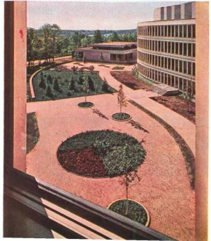
TRANSITION between modern building and rustic site (above) is softened by gentle curve of walls and subtle tint of the windows. Rib effect created by adjoining window frames gives vertical texture to walls, offsets emphatic horizontal spandrel lines.
