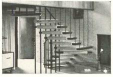
Architect J. Herbert Brownell designed this attractive stairway. Treads, composed of 3-inch thick laminated wood, are suspended on one end from 3/8-inch diameter steel rods, and on the other end by 3-inch diameter pipe columns. The upper ends of the rods are welded to the bottom of one of a pair of 10 WF 15 beams which support the balcony.
