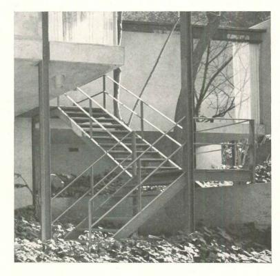
Thin lines of steel enhance the entry to this house designed by Craig Ellwood. The all-welded steel stairway is made up of small stock sections of structural shapes. Treads are of 14-gage sheet.
