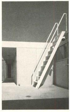
Reflecting the nautical atmosphere of the San Francisco Bay Area, steel ship ladders are used in this house to connect the upper level to a sundeck on the roof. The ladders are welded steel plates, with 1½-inch square steel tubes used as railings. Architect was Rolf Eiselin.
