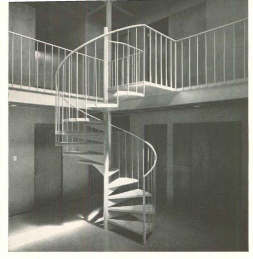
Two levels opening on a central court are connected with a spiral steel stairway in this home designed by architects Nelsen & Sabin. Treads, hanging from steel bars, are set into triangular frameworks of light steel angles.
