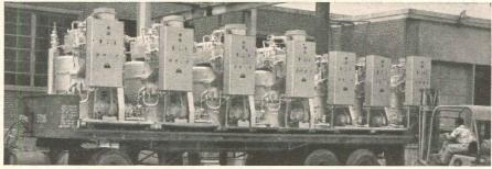
Small enough for seven boilers (total 835 HP) to fit on one truck
