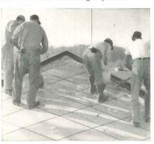
Lightweight "Incor" concrete roof slab is cast and finished over reinforcing.
