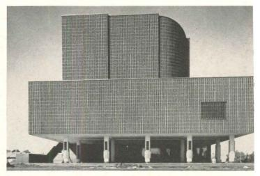
Exterior veneer of recently completed civic center consists of blue tile semi-circular in section. This material is also used on corridor walls. Lighting in meeting room is elegant, yet informal as shown in photograph on opposite page
