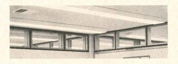
Centrally conditioned air is ducted to ceiling diffusers. High window strips give a feeling of spaciousness and eliminate distractions. Refrigeration is provided by two Carrier Automatic Absorption Machines powered by low-pressure steam which also supplies heating.
