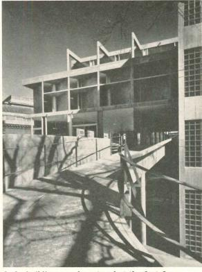
Curved element in foreground overhangs terrace partially screened by wall. Vertical slats admit light on north face but wall becomes continuous as it curves to the west. The directors studio workshop overlooks a planted terrace at the penthouse level, roof of curved foreground element will also be a terrace. Brises soleil are set at a 30 degree angle to screen the studio workshop from the late afternoon sun
