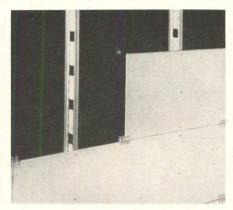
with studs spaced 24 in. on center. Sound transmission loss rating is given as 45 decibels. *National Gypsum Co.*, *Buffalo 2*, *N.Y.*
