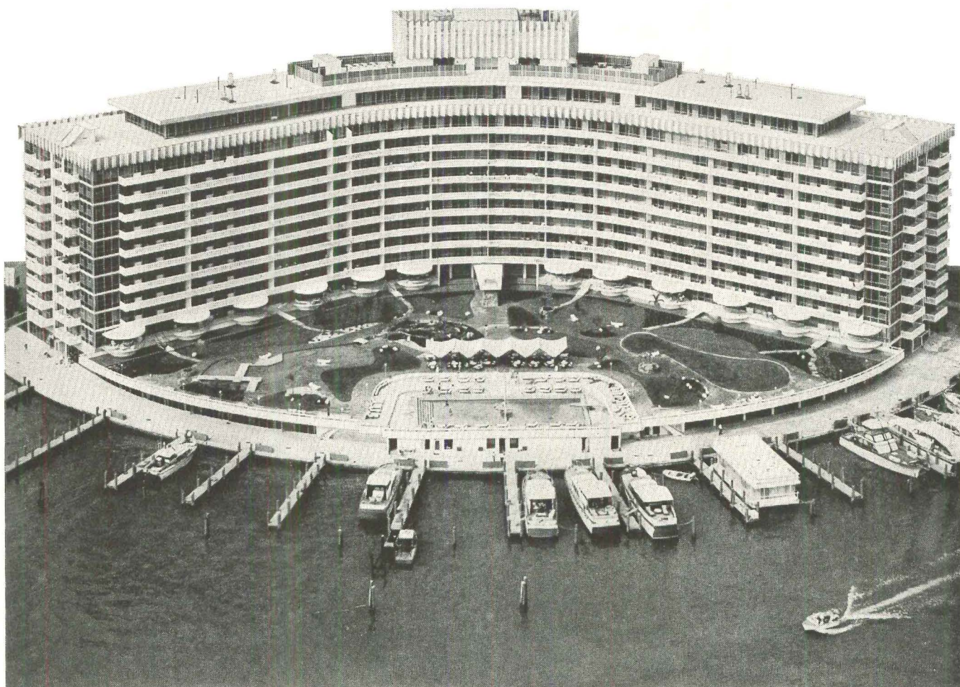
The King Cole was completed last fall. This photo clearly shows the variety of attractive architectural effects that have been accomplished with concrete.
