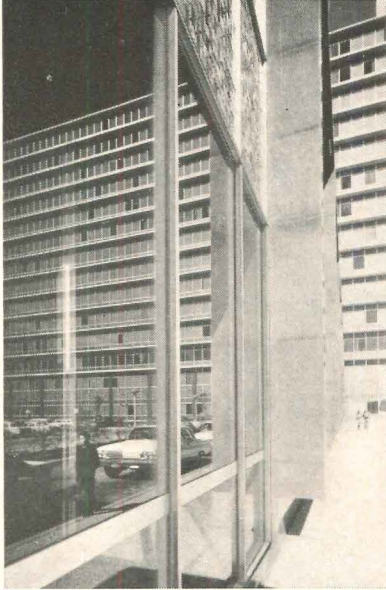
Detail photograph of Pittco 82-X Curtain Wall. Clean, crisp members show no visible fasteners—accept glass and mosaic spandrel panels without modification. Note distinctive reflective quality of PPG SOLARGRAY Plate Glass.
