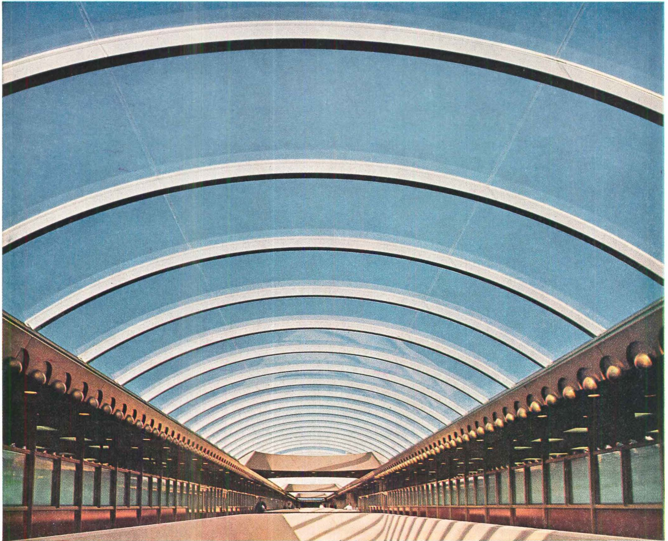
A soaring arch of Plexiglas admits natural light into mall areas of the Marin County Civic Center building. Frank Lloyd Wright, Architect; Taliesin Associated Architects of the Frank Lloyd Wright Foundation; William Wesley Peters, Chief Architect; Aaron G. Green, AIA, Architect Associated.
