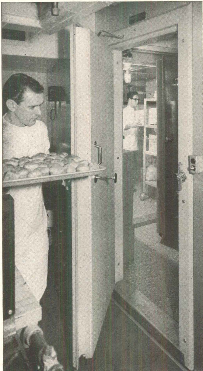
EASY OPENING Jamolite plastic doors facilitate rapid movement between kitchen area and cold room.
