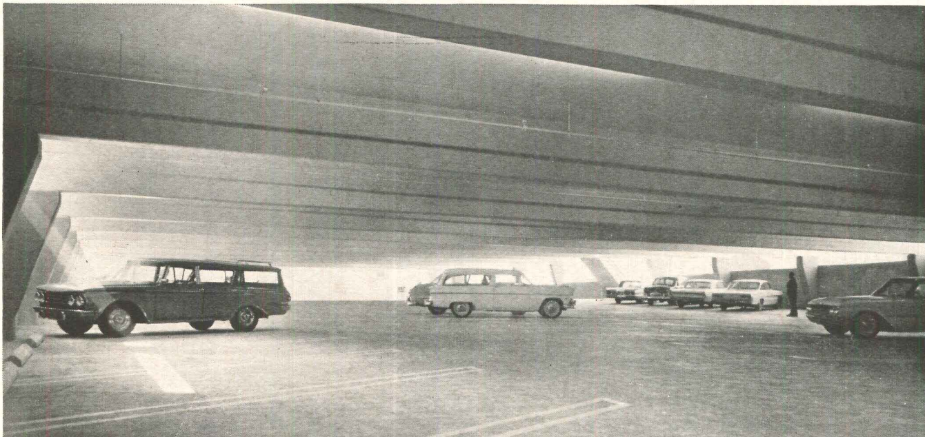
PARKING STRUCTURE AT WESTWOOD VILLAGE, CALIFORNIA • ARCHITECT: CHARLES M. BOLDON, AIA • ENGINEER: T. Y. LIN & ASSOCIATES INTERNATIONAL
