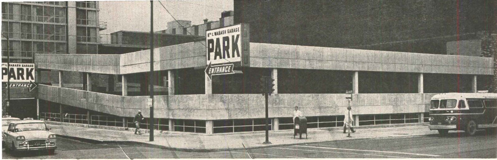
8th and Wabash Corporation Parking Garage, Chicago. Designed by Miller Engineering Company; built by Stuparitz Construction Company; both of Chicago. Area: 65,000 sq. ft.
