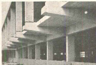
Lateral beams at second floor cantilever 7'-3".
