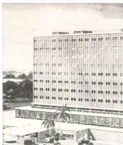
Mobile General Hospital, Mobile, Ala. Thomas Cooper Van Antwerp — Archt. Mobile, Ala. Manhattan Construction Co. of Texas — Contr. Houston, Texas
