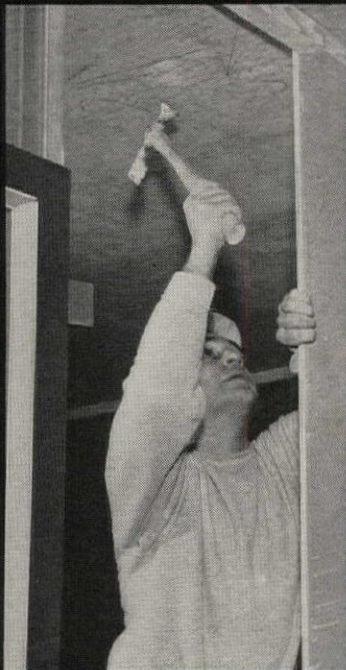
1. Nail face layer to ceiling and floor runners
