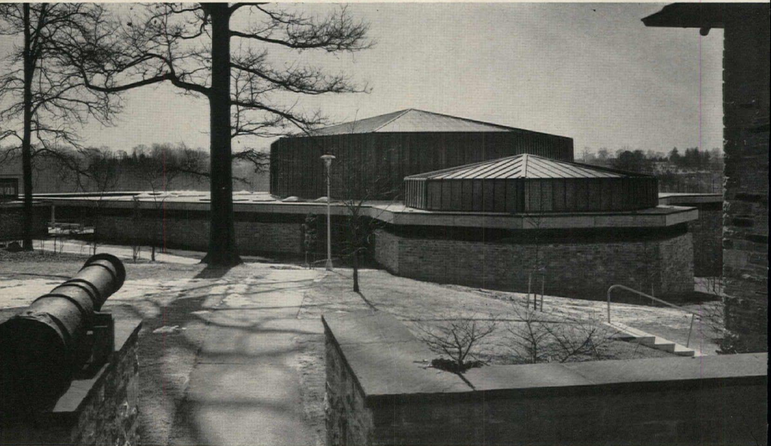
View from upper campus. Octagonal lecture hall in foreground. Roofs of both auditorium and lecture hall are covered with copper. Flat roof encloses auditorium lobby and exhibition area
