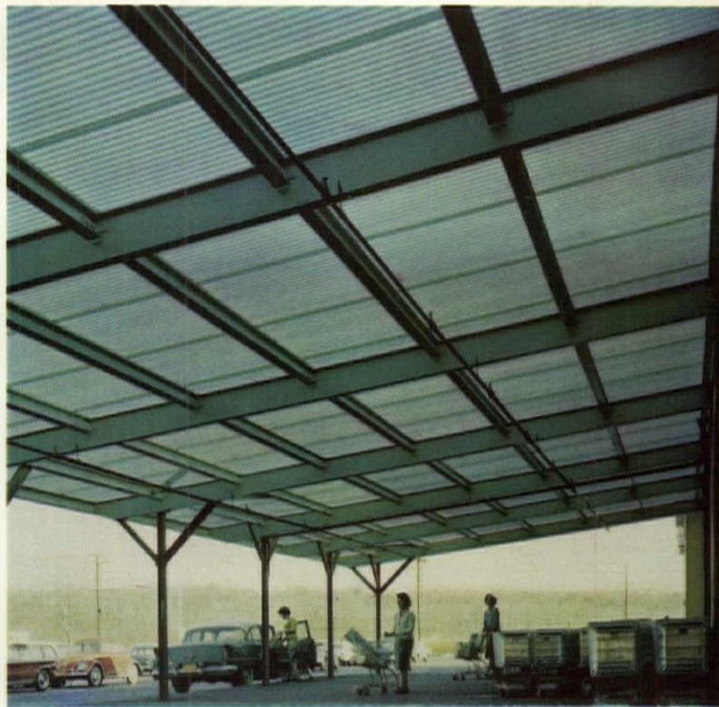
Long Island shopping center canopy provides all-weather protection.
