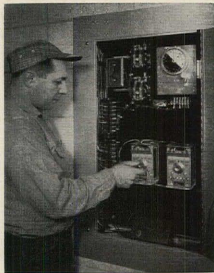
Wall-mounted box contains slab heating controls. Operation is programed by timer (T) which turns on power before start of school and off before dismissal. When slab temperature is below set point, control applies power to relay
