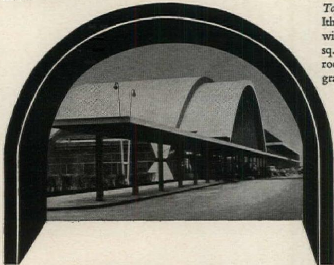
Jet-age cover —This ageless Overly parabolic roof covers an area of 26,000 sq. ft. at Idlewild Airport's International Arrivals Building. Crafted in enduring stainless steel, it will still be in service when tomorrow's planes are obsolete. Architects: Skidmore, Owings and Merrill, New York, N. Y.
