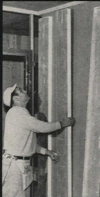
2. Apply adhesive-coated gypsum studs
