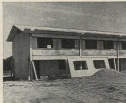
Roof units provide an overhang and built-in gutter. Roof and side wall units are 4" thick. Party walls are 8" thick and second floor slabs are 5" thick.
