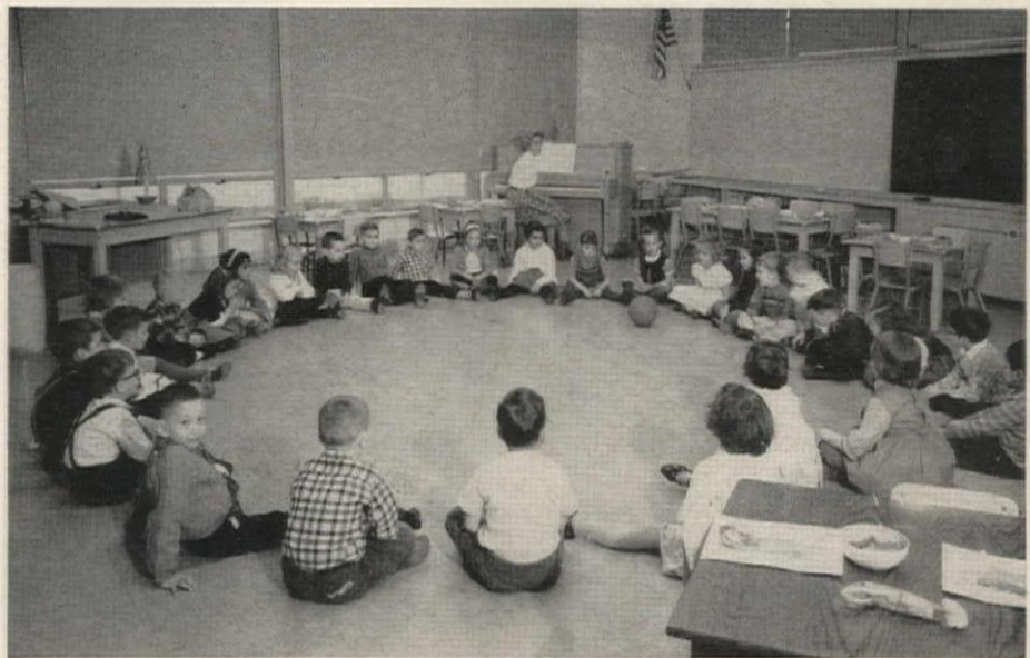
Children can sit comfortably on the floor even at zero degree outside temperatures. Slab is electrically heated to a temperature of 3 F below that of the room air
