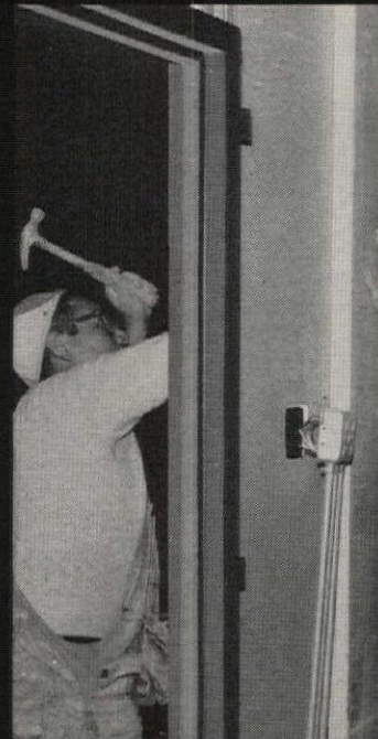
3. Secure gypsum studs with nails or screws
