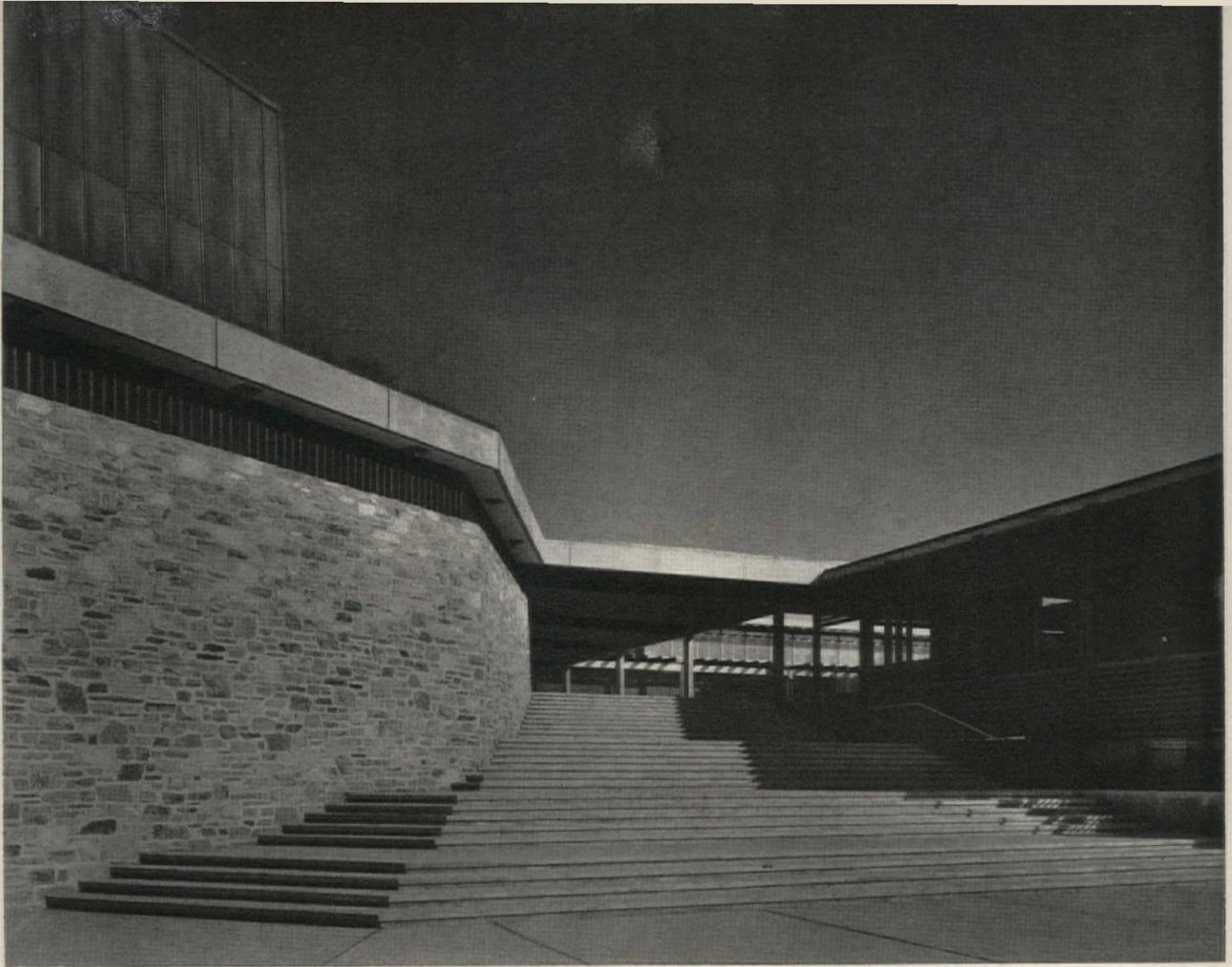
Stairway to upper campus. Courtyard to right at top of the stairs
