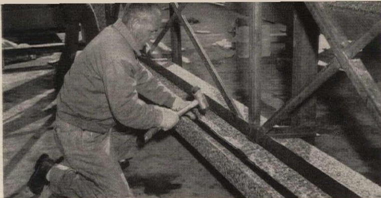
Neoprene gasket is wedged into the reglet of the precast frame
