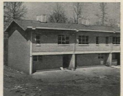
Buildings vary in size providing from four to sixteen dwelling units each. Exterior walls have masonry veneer. Note roof vent screens atop each unit.
