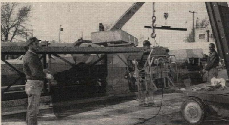
Sheet of bronze-color. Solar-reducing glass is next set in gasket slot
