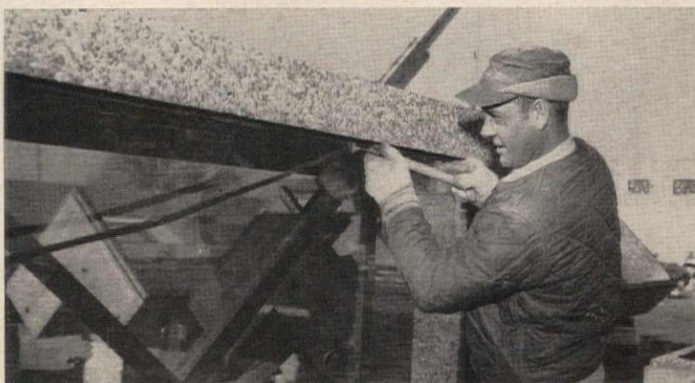
Neoprene zipper insert makes gasket form a tight seal around glass
