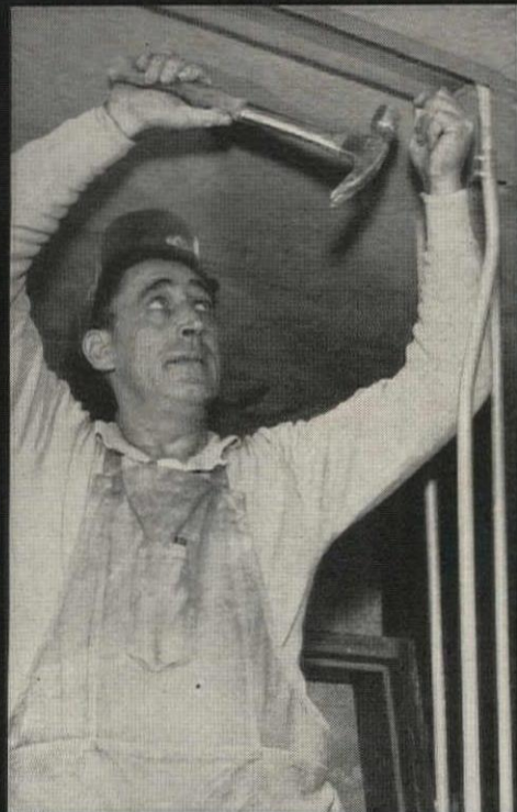
A. Install metal floor and ceiling runners
