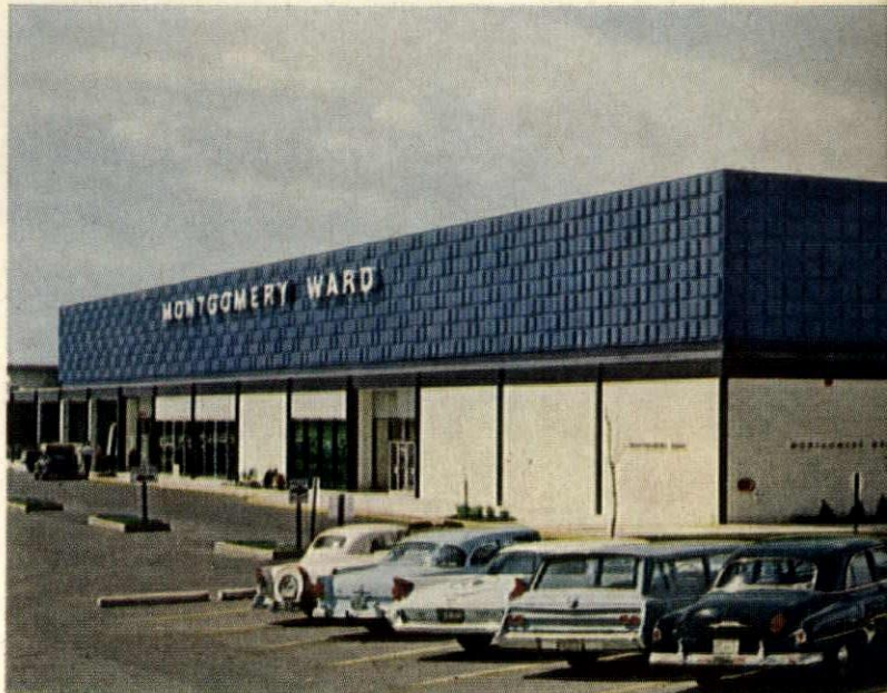
Montgomery Ward store, Apache Plaza Shopping Center, St. Anthony Village, Minn. Architects: Thorsen & Thorshov, Inc., Minneapolis, Minn.
