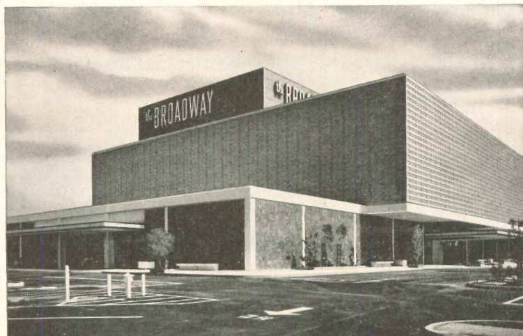
Broadway Department Store, West Covina, California. Chilled water for air conditioning is provided by a York Hermetic Centrifugal system. Building owner, New York Life Insurance Company. Architect, Charles Luckman & Associates, Beverly Hills, California. Structural Consultants, Brandow and Johnson, Los Angeles. Mechanical Consultants, J. L. Hengstler, Los Angeles. Mechanical Contractor, Cal-Aire Conditioning Company, Los Angeles. General Contractor, Steed Bros., Alhambra, California.
