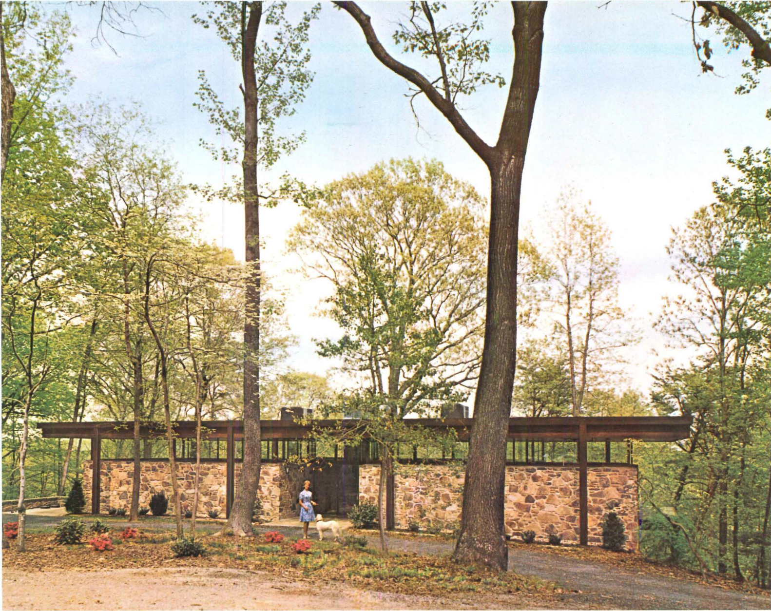
The weathered color of the exposed steel beams and columns blends harmoniously with the native stone and the surroundings of this Maryland residence.
