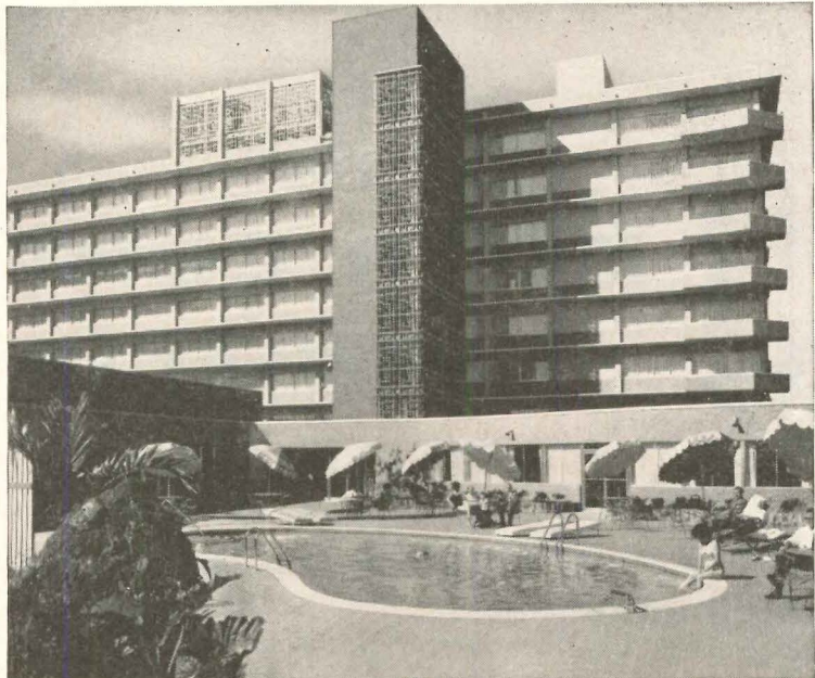
Continental-Houston Motor Hotel, Houston, Texas. 228 York Fan-coil units provide air conditioned comfort for guests of this motor hotel. Chilled water for cooling is furnished by two York Hermetic Turbopaks. Owner, Continental-Houston Motor Hotel Co., Inc. Builder, Manhattan Construction Co., Houston. Architect, William Hirsch, Los Angeles. Structural Engineers, Manhattan Industrial Corp., Houston. Mechanical Contractor, Barber Co., Inc., Houston. Mechanical Engineer, Roy F. Williams, Houston.
