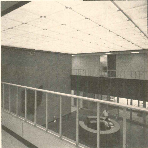
High above the lobby, Sylvania's Sylva-Lume System provides diffused, shadow-free illumination to the reception area below.
