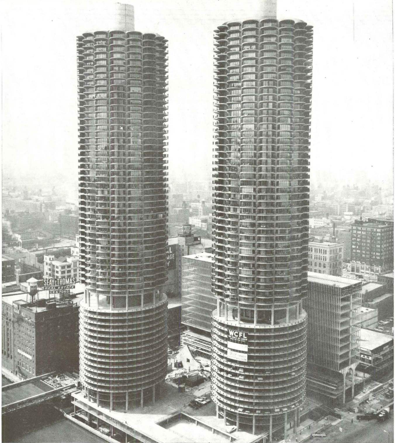
Marina City, twin 60-story apartment towers in Chicago. Architect, B. L. Goldberg, A. I. A.
