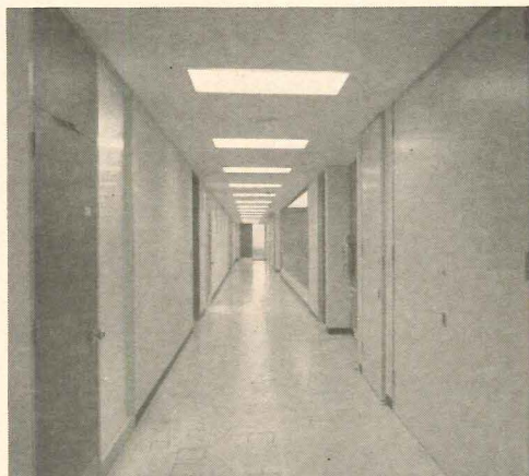
Well-lighted corridors also utilize Sylvania's Sylva-Flo Troffers.
