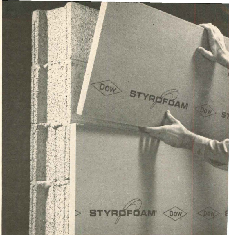
4. Press Styrofoam FR into place. It installs fast, stays dry for year-round comfort.
