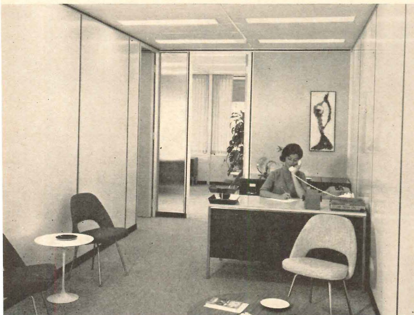
Office partitions have aluminum frames and plastic panels
