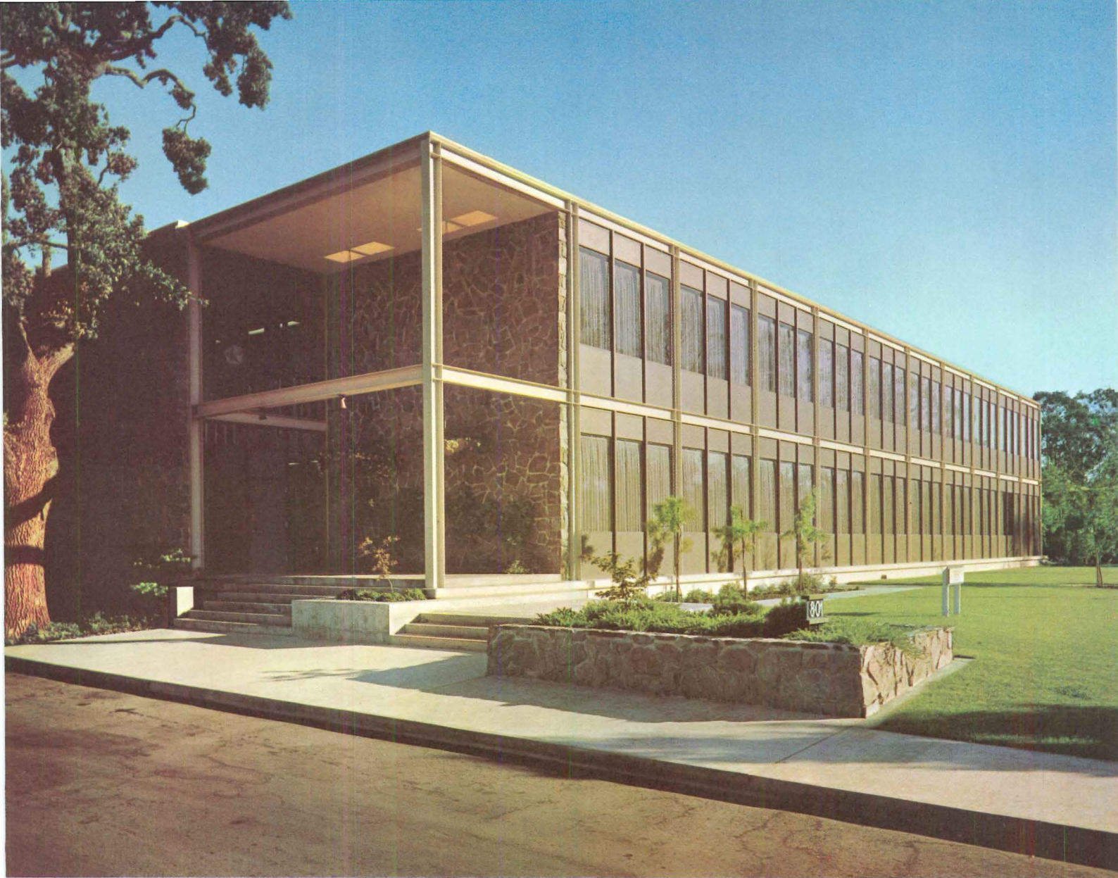
Weldwood #58 /AM umber Glasweld sandwich panels on the Demmon-Hunter Building, Palo Alto, California. Architect: Paul James Huston, Palo Alto, Calif. Installer: Fentron Industries, San Francisco.
