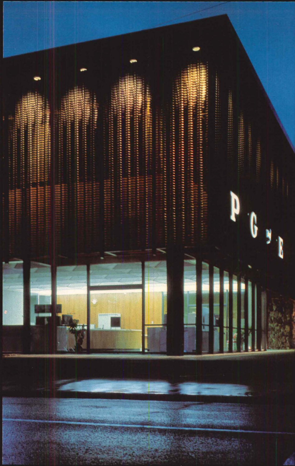
Pacific Gas & Electric Co., San Rafael, Calif. Carl F. Gromme and Ralph B. Priestley, AIA, Architects General Contractor: MacDonald, Young & Nelson, Inc. KALCOLOR® aluminum curtain wall: Kawneer Company, Richmond, Calif., Niles, Mich.
