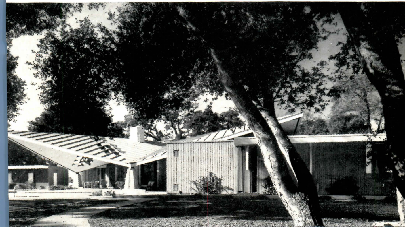
ing a point. Cantilever roof spreads its protecting wings over this tree- contribution to modern, comfortable living. The vertical wood g adds special beauty to the total concept. Architects: Anshen & Allen.
