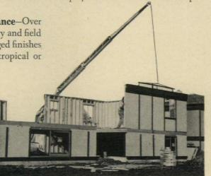
Wall section for this new house is lifted by boom crane and moved into position for installation. Interior wall is completed with foil-faced fiber insulation and 1/2 in. dry walls. Prefabricated walls are erected quickly and easily.
